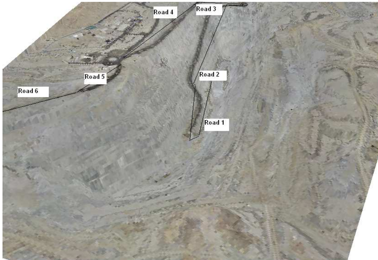
Figure 3.5: Some of the roads around the Rössing open pit (scale: 1:2500)
