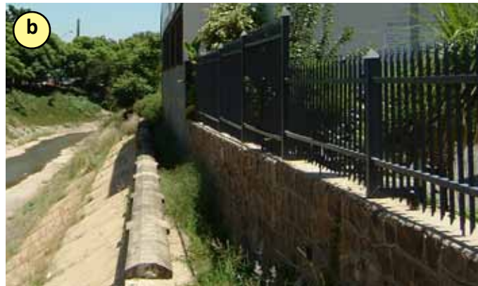
FIGURE 39. VIEW NORTHWARDS INTO THE CHANNEL - THE OLD ROCK WALL ON THE RIGHT WAS BUILT AS AN HYDRAULIC STRUCTURE AND RAISES THE GROUND LEVEL AT THE BMW MOTORCYCLE SHOP ABOVE THE TOP OF THE CHANNEL
