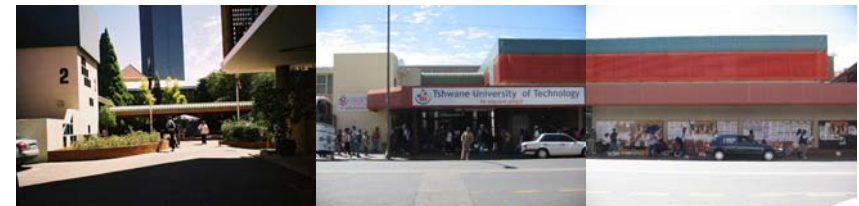
Fig.10.10: Building 4 – View of building from Nelson Mandela entrance to the campus
