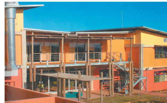
Figure 4.3 Timber & steel materials where carefully combined
