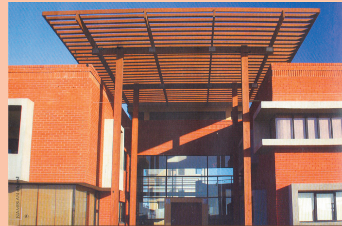
Figure 4.9: Entrance of the building
