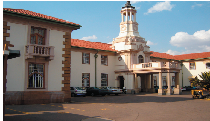
Figure 2.20: The administration block, heritage building
