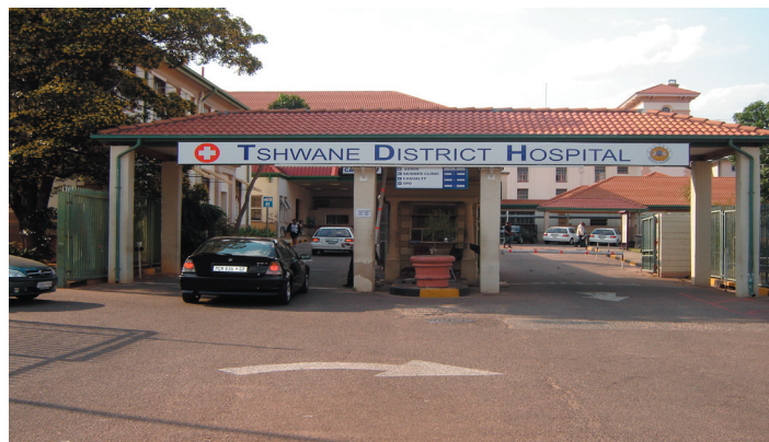
Figure 2.21: Entrance of the District Hospital
