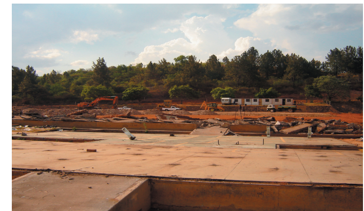
Figure 2.24: Northward view from the site
