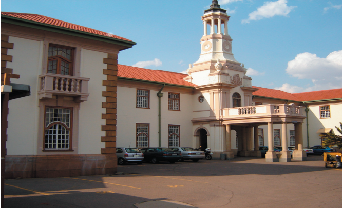
Figure 2.4: Old administration (Heritage building) Architect: John Cleland (DPW)
