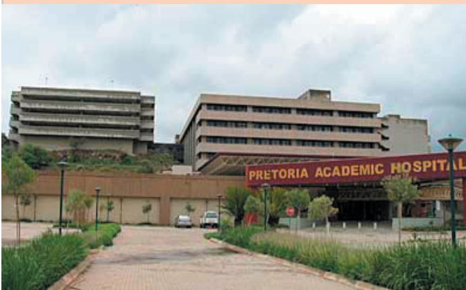
Figure 2.6: New Pretoria Academic Hospital Architects: Leap/MMA
