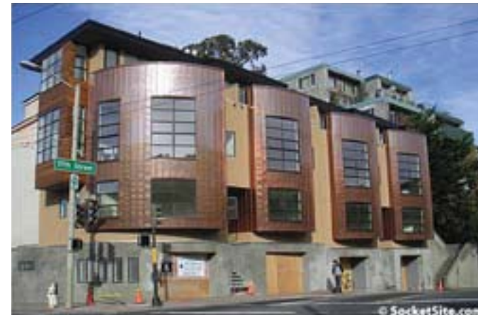
Figure 7-17. Newly installed shiny copper. h tp://www.socketsite.com/17th_and_clayton.html
