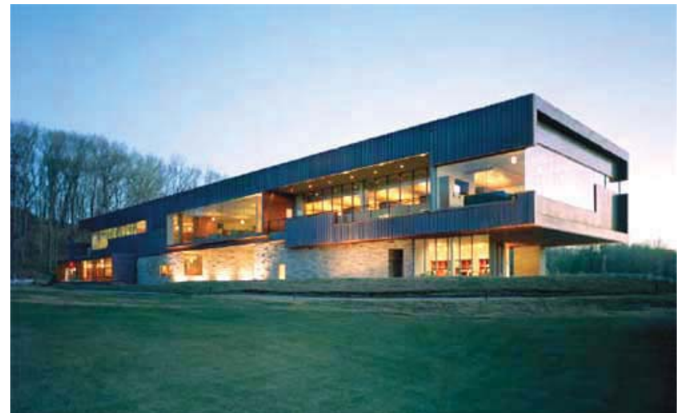
Figure 4-27. Photo of the Blessings Golf Clubhouse
