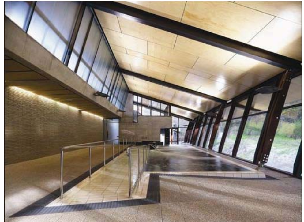
Figure 4-18. Photo of the Hepburn Springs Bathhouse
