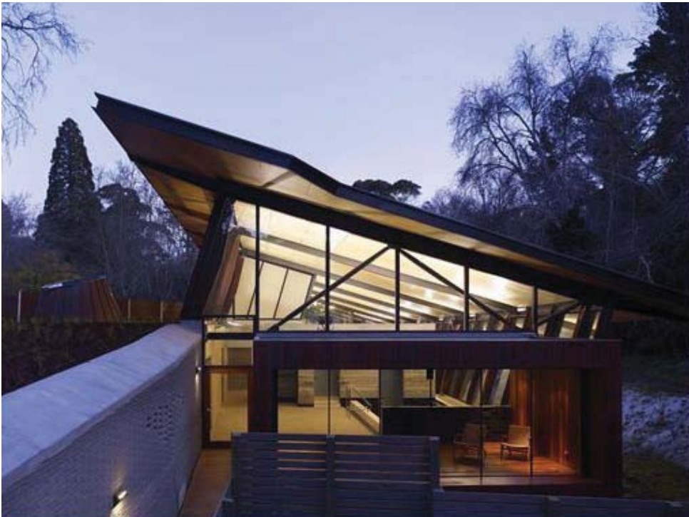
Figure 4-16. Photo of the Hepburn Springs Bathhouse
