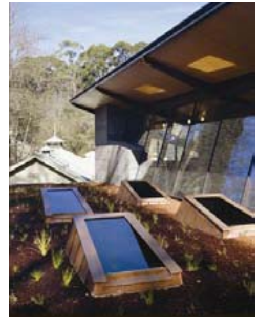
Figure 4-17. Photo of the Hepburn Springs Bathhouse
