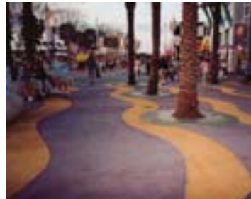
Figure 7-21. Example of colour stained concrete.
