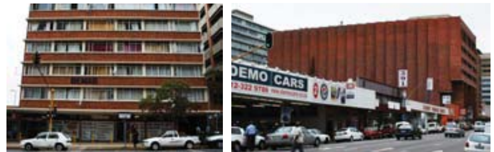
Figure 7-18. Photo's of dark concrete buildings surrounding the site. 7 | 125
