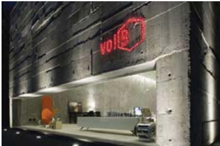
Figure 7-14. Example of concrete constructed in timber casting shutters. http://fazyluckers.com/
