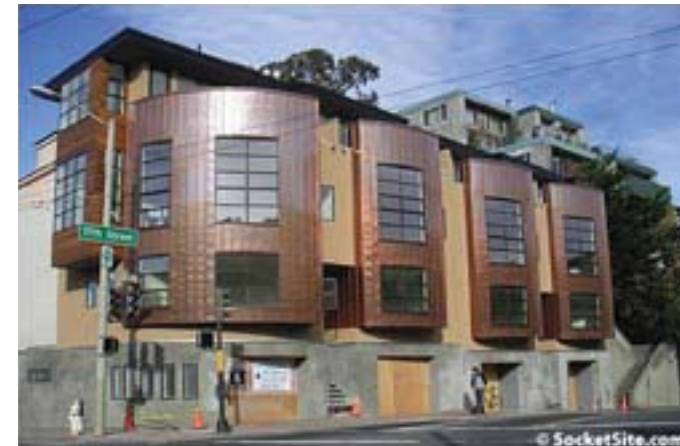
Figure 7-17. Newly installed shiny copper. h tp://www.socketsite.com/17th_and_clayton.html
