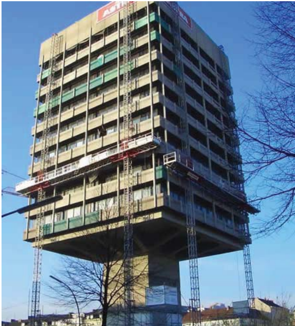
Figure 4-32. Photo of the Cantilevering tower Building
