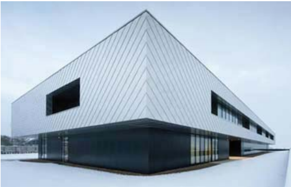
Figure 4-26. Photo of the Circle Bath Hospital
