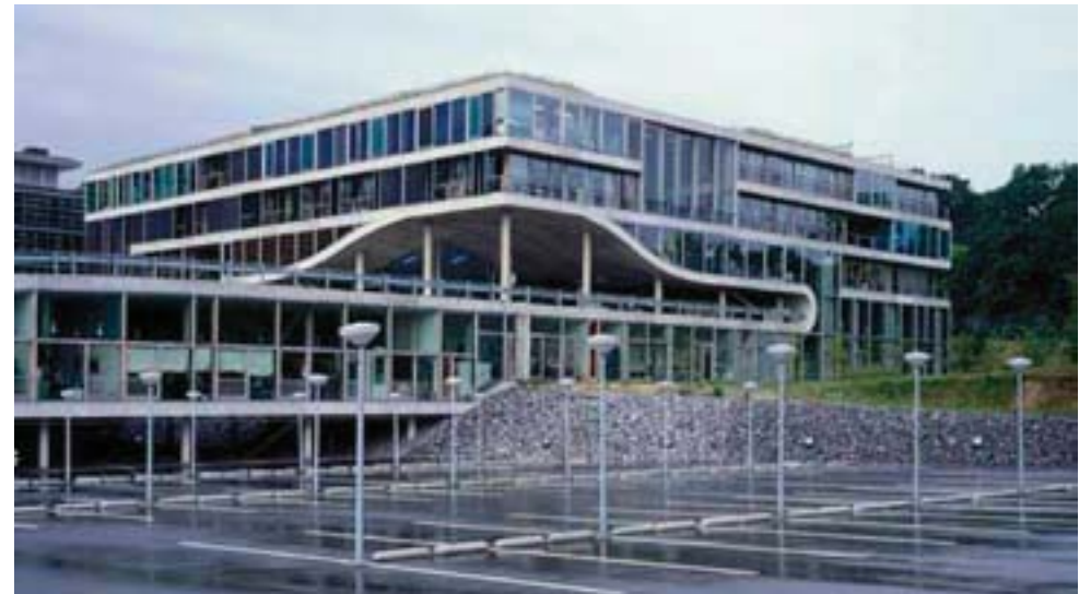
Figure 4-33. Photo of Villa VPRO
