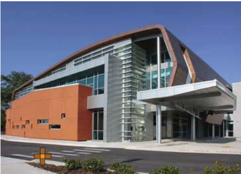
Figure 4-6. Photo of LaVilla Medical Office Building.
