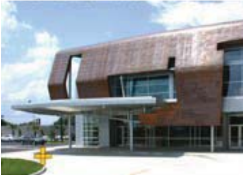
Figure 4-5. Photo of LaVilla Medical Office Building.
