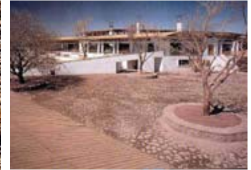
Figure 4-11. Photo of the Hotel Atacama Oasis.
