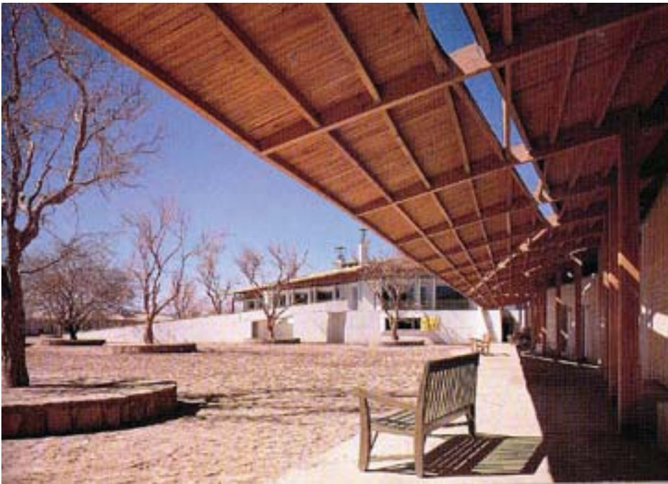
Figure 4-9. Photo of the Hotel Atacama Oasis.
