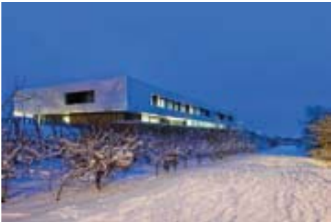
Figure 4-24. Photo of the Circle Bath Hospital
