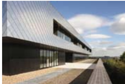
Figure 4-25. Photo of the Circle Bath Hospital
