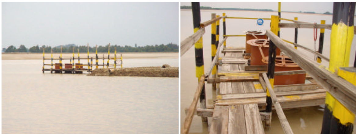
Figure 2.16: Decant tower at Mispah tailings dam
