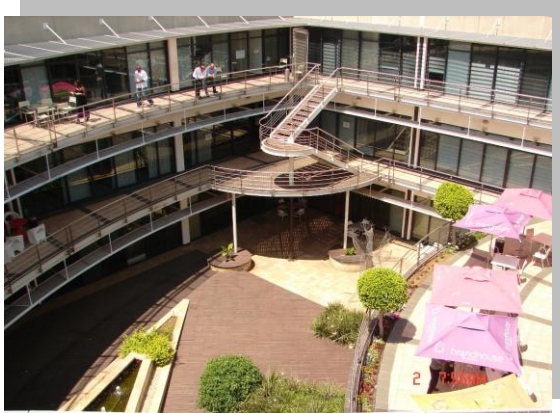
Figure 6: Private square inside office building
