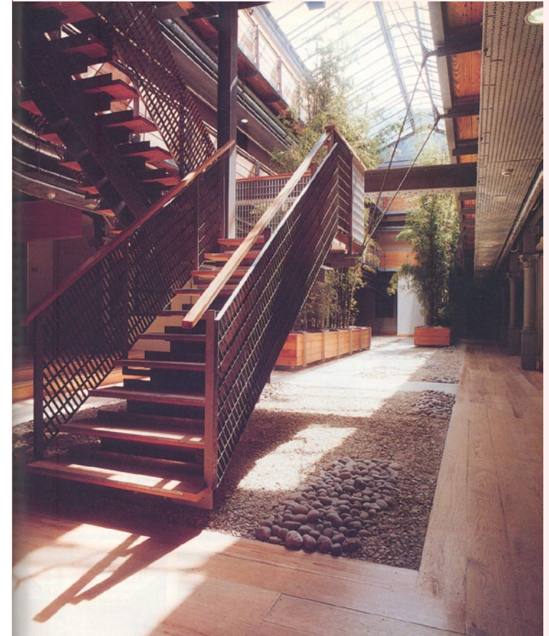
Fig. 5.91. The atrium in the Smithfield Buildings.
