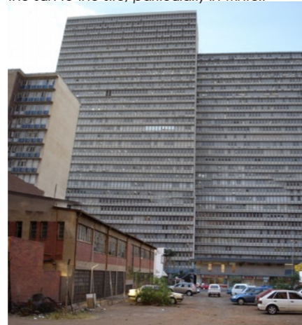
Fig. 5.8. The Poynton Building blocks out most of the sun to the site, particularly in winter.
