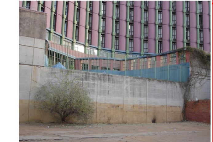
Fig. 5.9. Rear view of the HSRC Building. The design needs to connect with the courtyard 2 850mm above ground level and the basement parking 450mm below natural ground.
