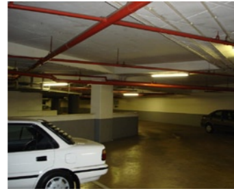
Fig. 5.10. Interior of the HSRC parking garage.
