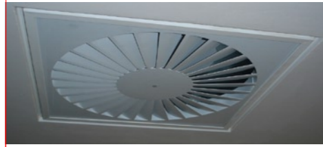
Fig. 2.15. An airconditioner diffuser can be used to generate grey noise at the required level.
