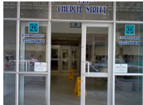
Fig. 2.19. Access control at neighbouring buildings.
