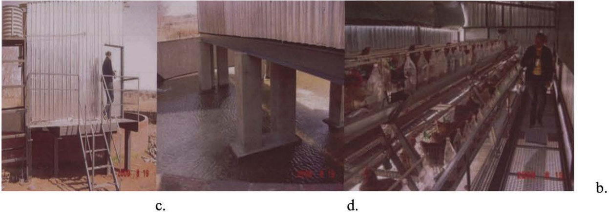
Figure 3.2 a. Chicken house constructed over fish dam b. Front view c. Dam underneath the chicken house d. Inside view
