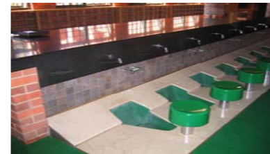
(Left: Fig. 23. Dar-as-Salaam Mosque, Laudium, South Africa, 2002, indicating the individual cellular trays in the ablution area).
