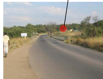
(Fig. 40. The site in context). View 8: View of bridge over Crocodile river
