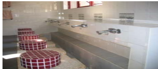
(Left: Fig. 20. Brits, Friday Mosque, 1995, indicating the seating and channel system in the ablution area).
