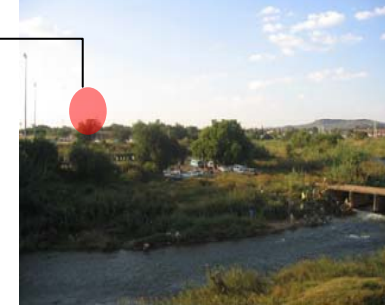
(Fig. 44. The site in context). View 9: Smaller pedestrian bridge behind community center
