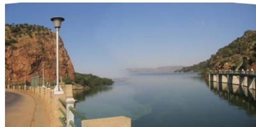
Fig. 9. Brits in general. Panoramic of Hartebeespoort Dam from bridge
