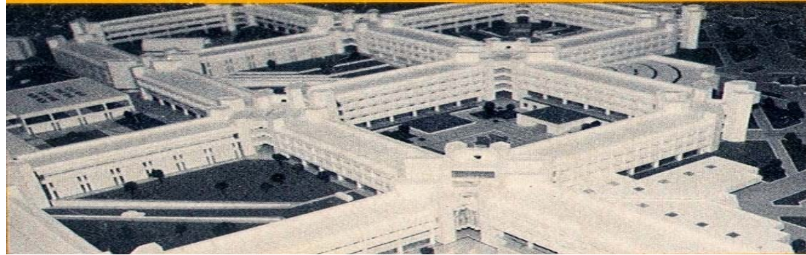
(Fig. 107.). Government administrative centre, Riyadh, Saudi Arabia. (Picture from Lari: 1990, p.90).
