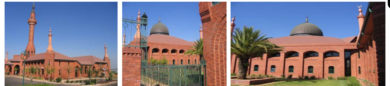
(Fig.'s 18-20). Dar-as-Salaam, Laudium, 2002 – celebrates a 'wall-architecture' decorated by a face-brick façade, with recessed windows informed by the internal requirements of the Mosque.
