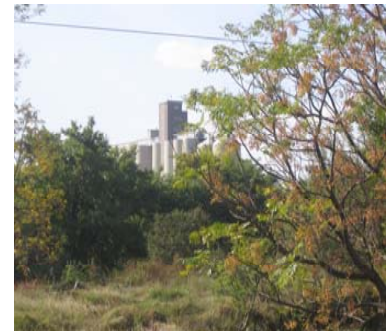
Fig. 65. View from southern side towards granaries
