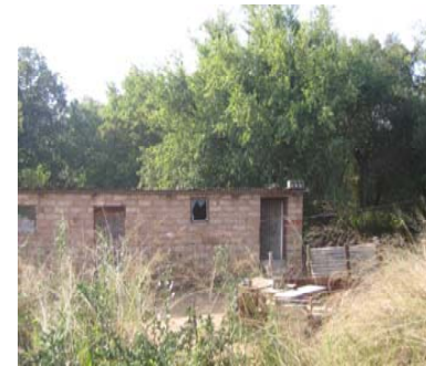
Fig. 66. Existing house on site built from local low-intensity river-sand-concrete blocks
