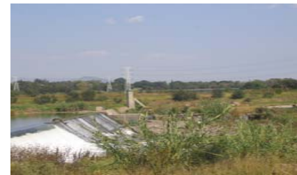
Fig. 77. Close-up of waterfall at reservoir
