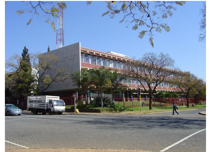
Fig 13. View of fire brigade to the west of the site across Bosman Street
