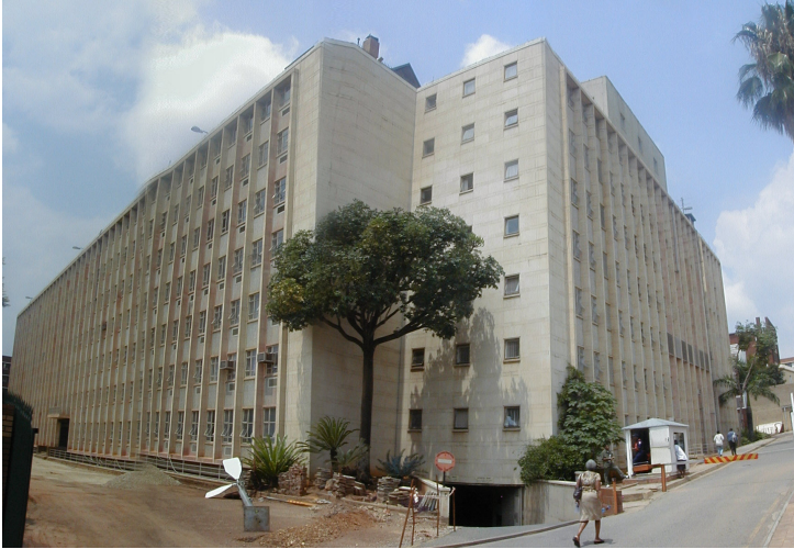
Fig 9. NZASM building on the east boundary of the site
