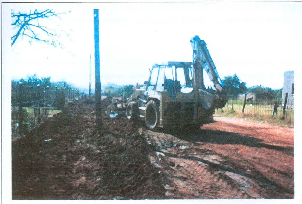
Plate 3: Construction site at Vlaklaagte: A scene for observation
