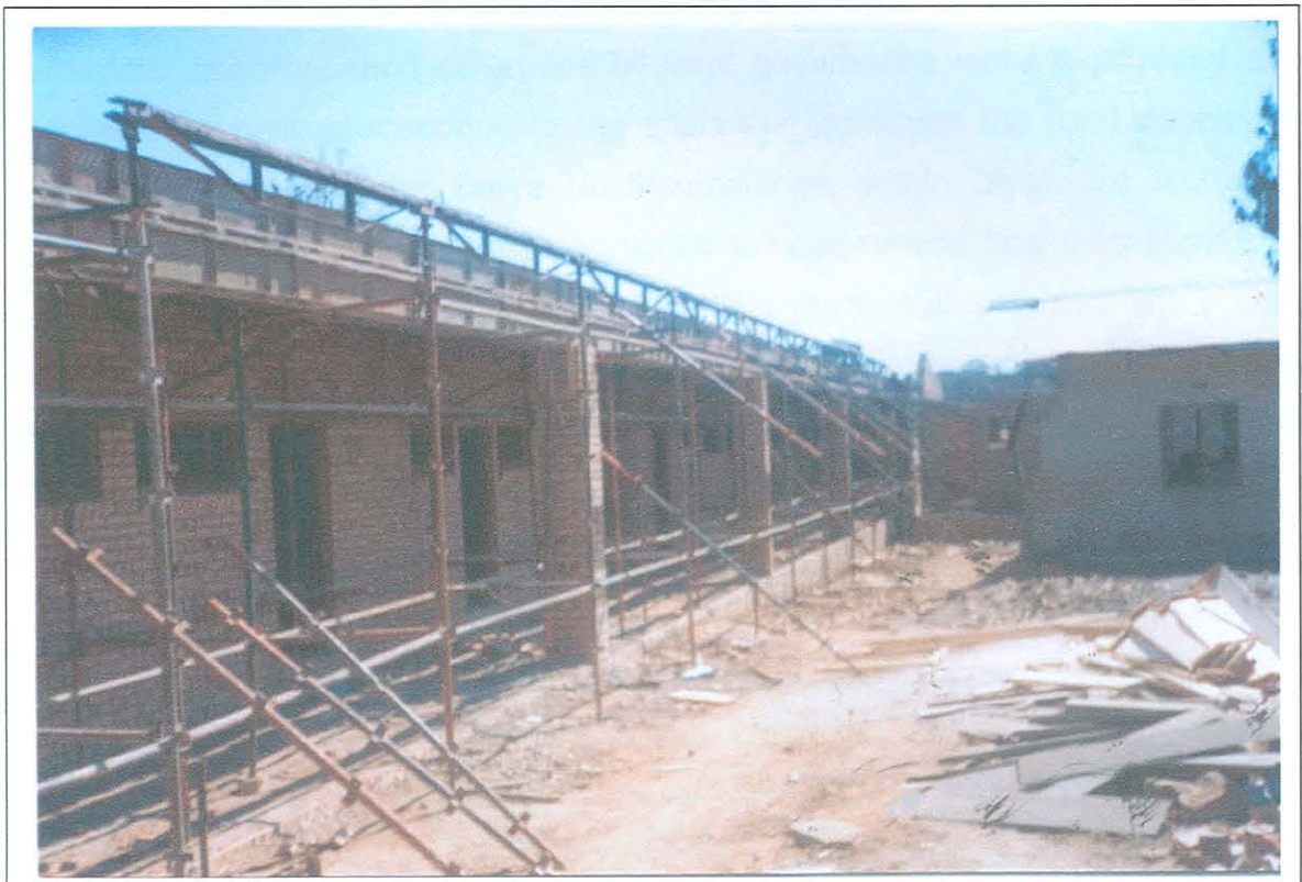
Plate 2: New school being erected at Ntwane (Moutse), 2000
