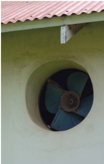
Fig.84 - Ventilation fan, existing architecture
