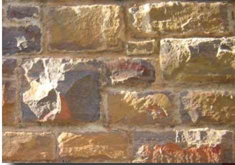
Fig. 60 - Stone of old retaining wall
