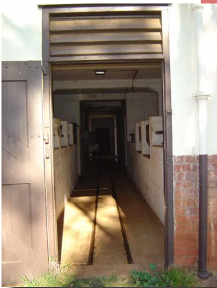
Fig. 53 - Steel cocopan track as seen from end of building
