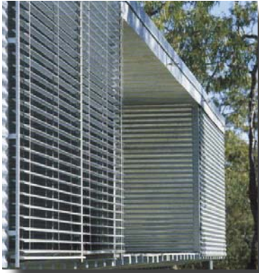
Fig. 75 - Adjustable louvres used together with corrugated iron
