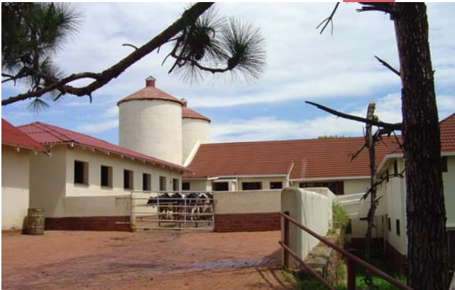
Fig. 19 - Eastern view of the old stable buildings
