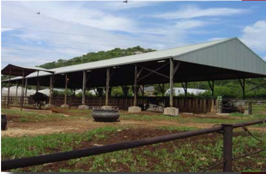
Fig. 22 - Steel cattle shelter
