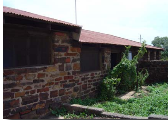
Fig. 20 - Exterior view of stone cattle housing
