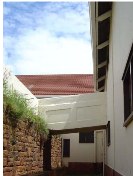
Fig. 54 - Stone retaining wall behind main building
