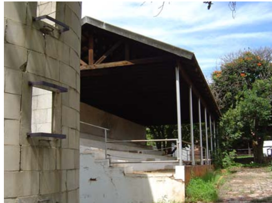
Fig. 21 - Small pavilion to the side of the cattle shelter
