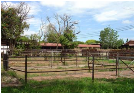
Fig.88 - South end site structures
