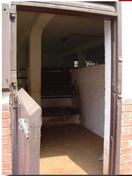
Fig. 52 - Concrete columns and beams as seen from outside
