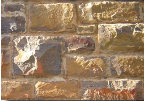
Fig. 60 - Stone of old retaining wall
