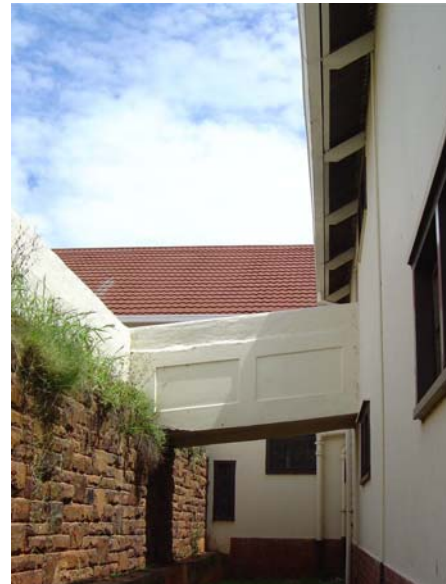
Fig. 54 - Stone retaining wall behind main building
