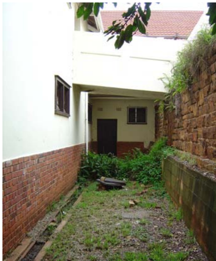
Fig.86 - Area between retaining wall and back wall of building
