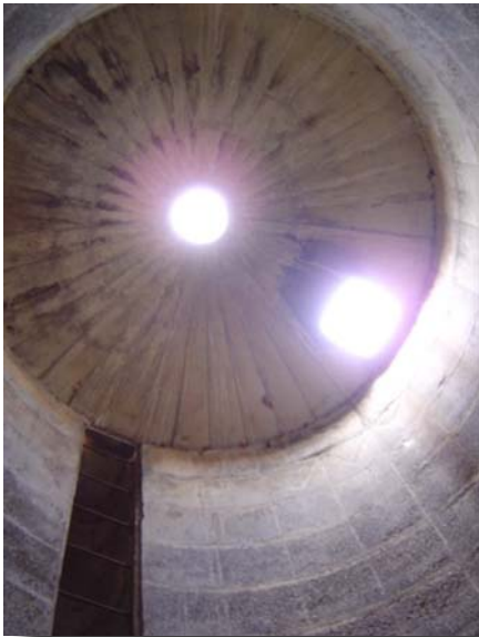
Fig.81 - Inside of silo
