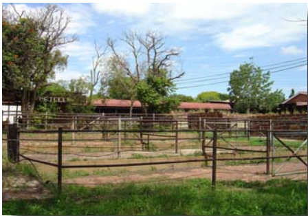
Fig.88 - South end site structures
