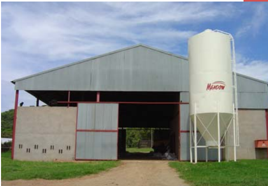
Fig. 23 - Equipment and feed storage shed
