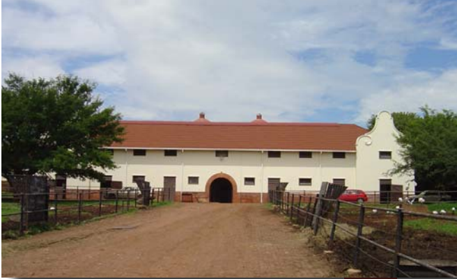
Fig. 18 - Front view of the main old stable building
