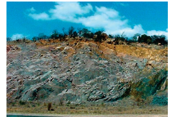
Figure 4.9 Portions of the landscape are cut away for road construction exposing the crude texture of the rock. This is sighted specifically in the Waterberg mountain range en route to Makhado
