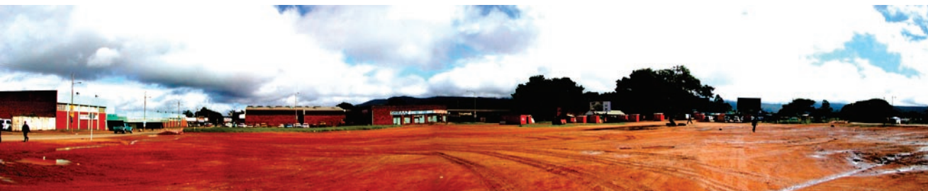
Figure 4.18 Below: Red sand at the bus depot
