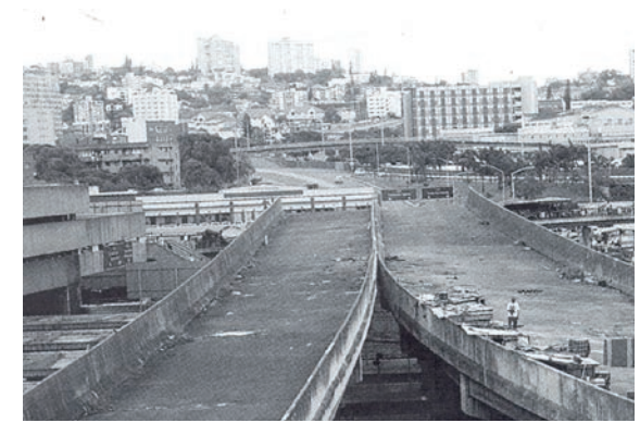
Figure 3.14: View of the abandoned highway before occupation by the Herb Traders
