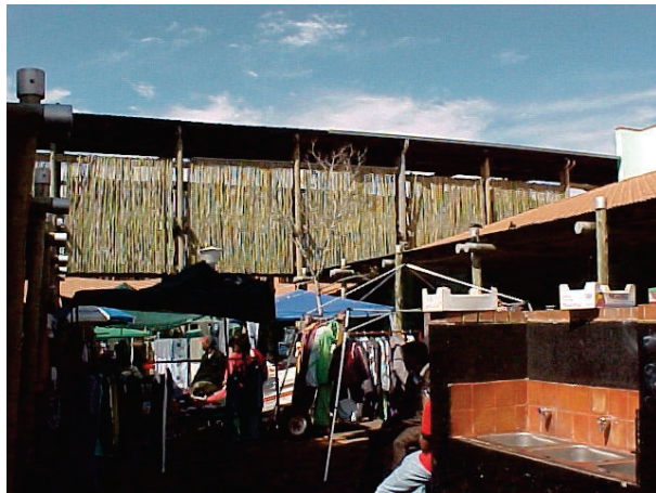
Figure 3.41. View of courtyard walls made of lathes
