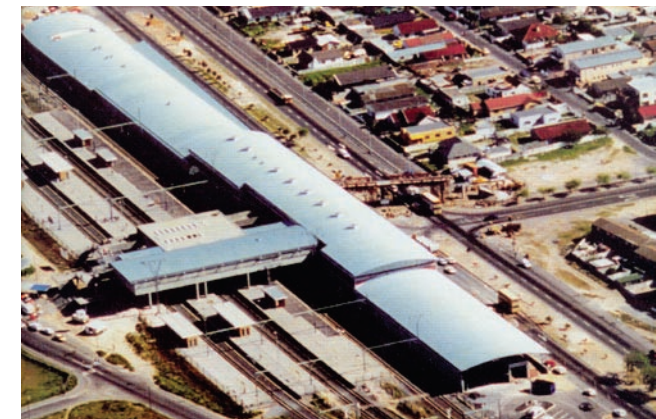
Figure 3.3 Aerial photograph of the complex, showing roof as enclosing element
