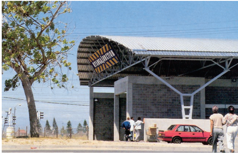
Figure 3.4 The simply detailed structure encloses the concrete block and frame buildings
