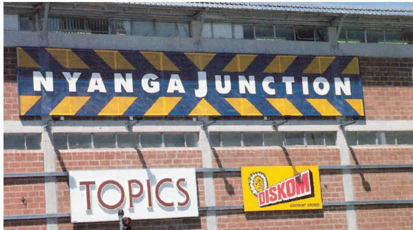
Figure 3.2. Advertisement boards fixed to steel tubing
