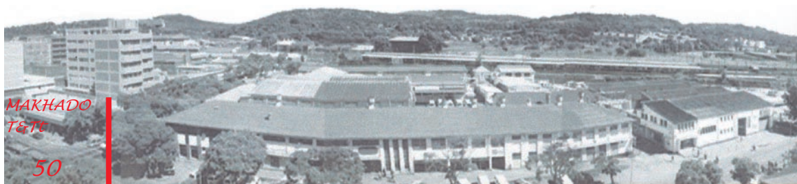
Figure 3.31. Photograph of Dairy Mall from the fire station
