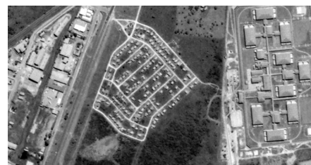
Figure 1.20 Prison housing placed adjacent to N1 Highway
