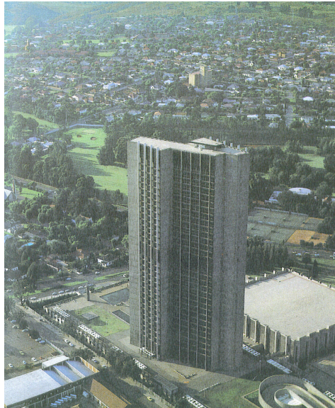
Figure 14: Broadcasting Centre, Auckland Park, Johannesburg. Source: SABC, Annual Report , 1981, p.115.
