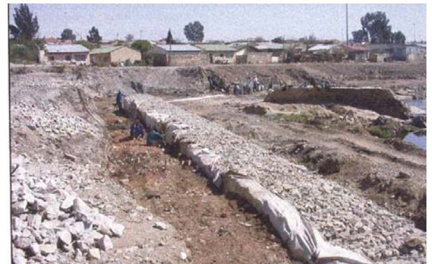
Figure 68 Gabions works at the Jukskei River. About 2/3 of the stabilizing work in the river is already completed. The next phase of implementation includes the area which is bordering with the site. (Source- ARP infrastructure)
