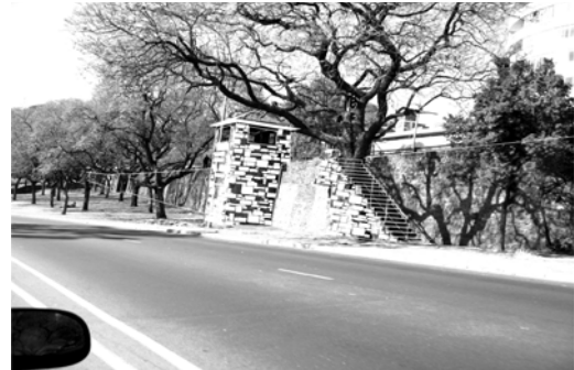
07.11. Louis Botha Stone retaining wall
