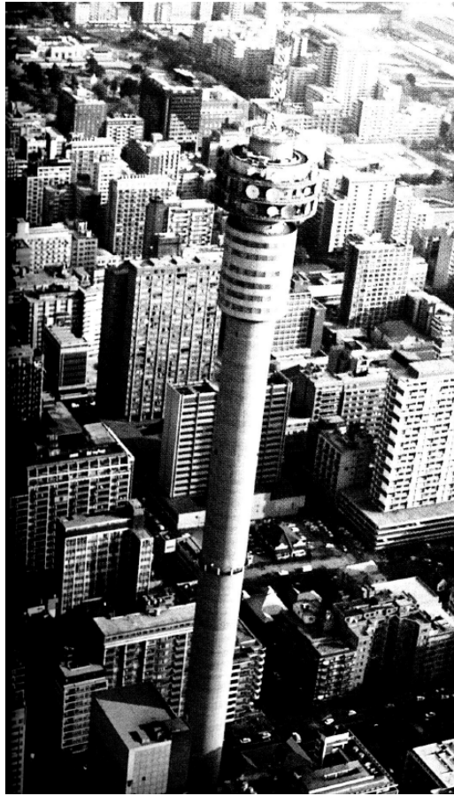
02.32. The Hillbrow communications tower
