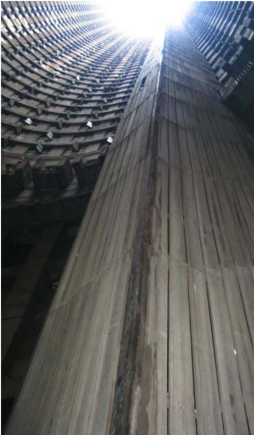
02.36. Inside the Ponte tower: elevator shaft
