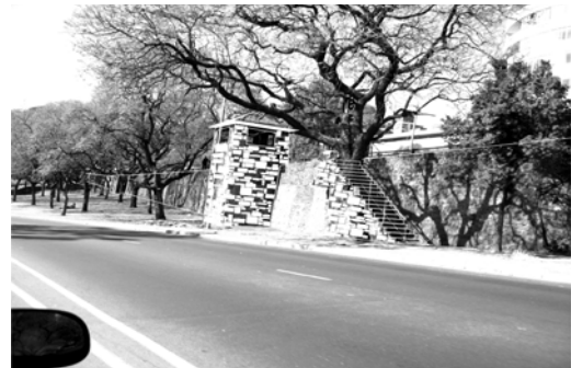
07.11. Louis Botha Stone retaining wall
