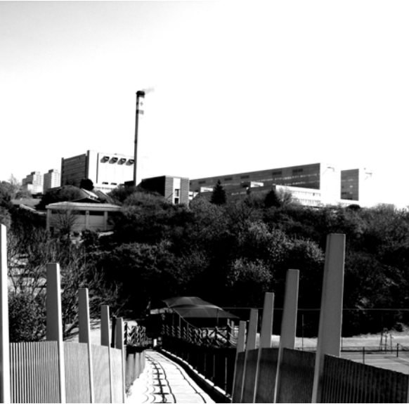
07.4.2. View of from st Johns pedestrian bridge to johannesburg general hospital
