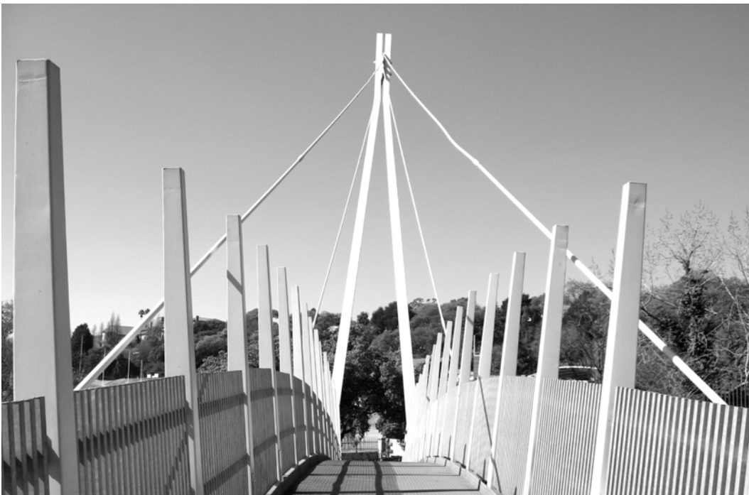
07.36. St Johns - Roedeaan pedestrian bridge
