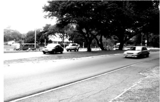
07.08. View of intersection B
