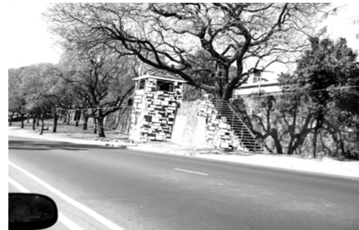
07.11. Louis Botha Stone retaining wall
