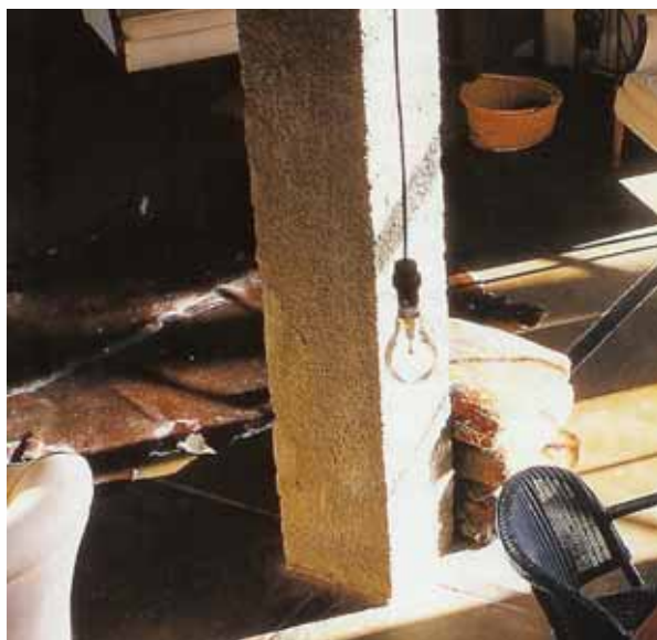
1: Column structure: exposed concrete
