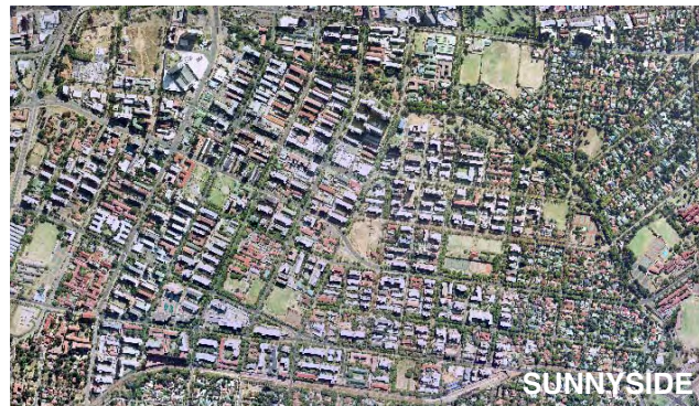
Illus. 13: Aerial photo of Sunnyside. [GIS UP, 2005]
