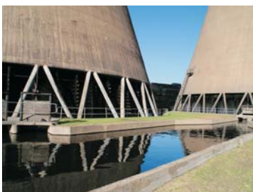
fig 5.7 Water channel leading to cooling towers
