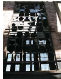
fig 5.22 Power station: derelict
