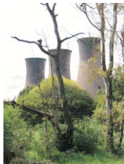
fig 2.2 Cooling towers viewed from Quagga road
