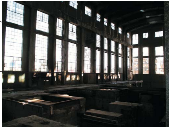
fig 5.21 Turbine Hall Johannesburg
