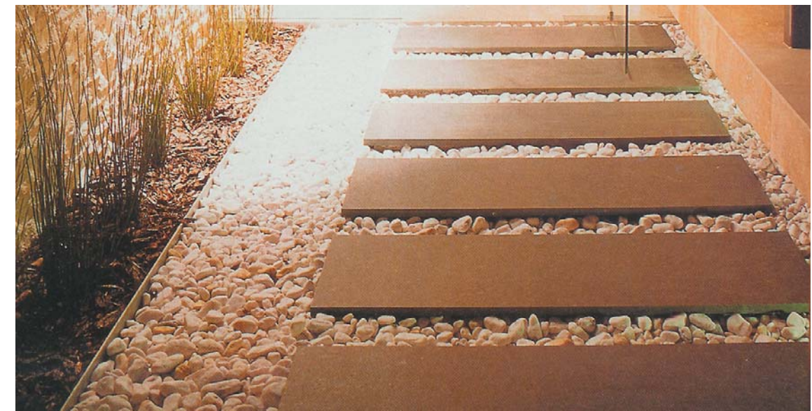
fig. 5.10. Cast concrete pavers on gravel
