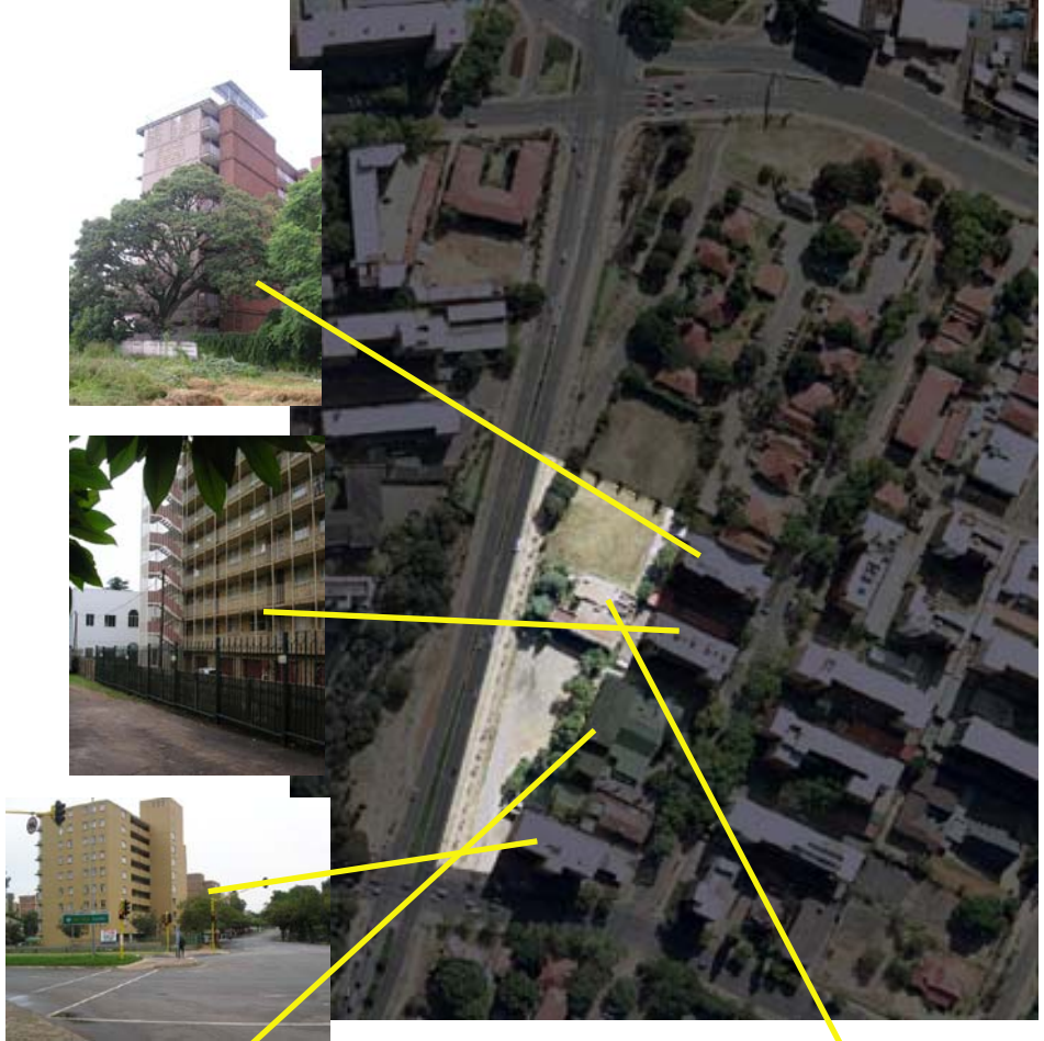
aerial photo of site 2005
