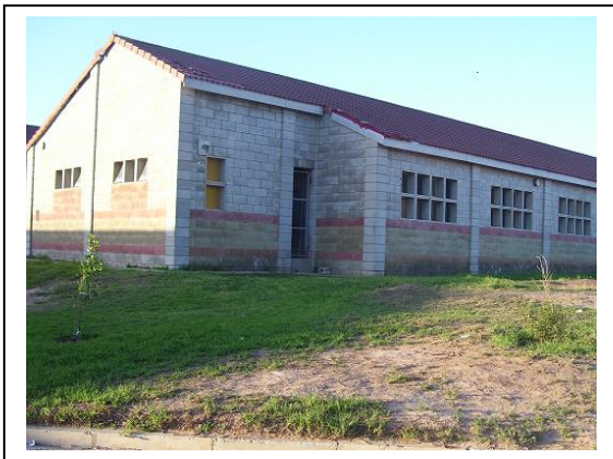
PHOTOGRAPH 3.1: The primary school
