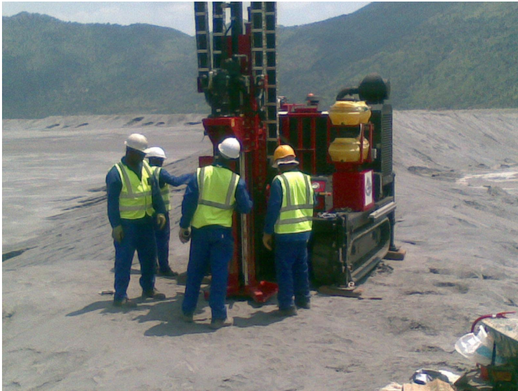
Figure 21: Direct push probe drilling on the tailings storage facility on 20 February 2012.
