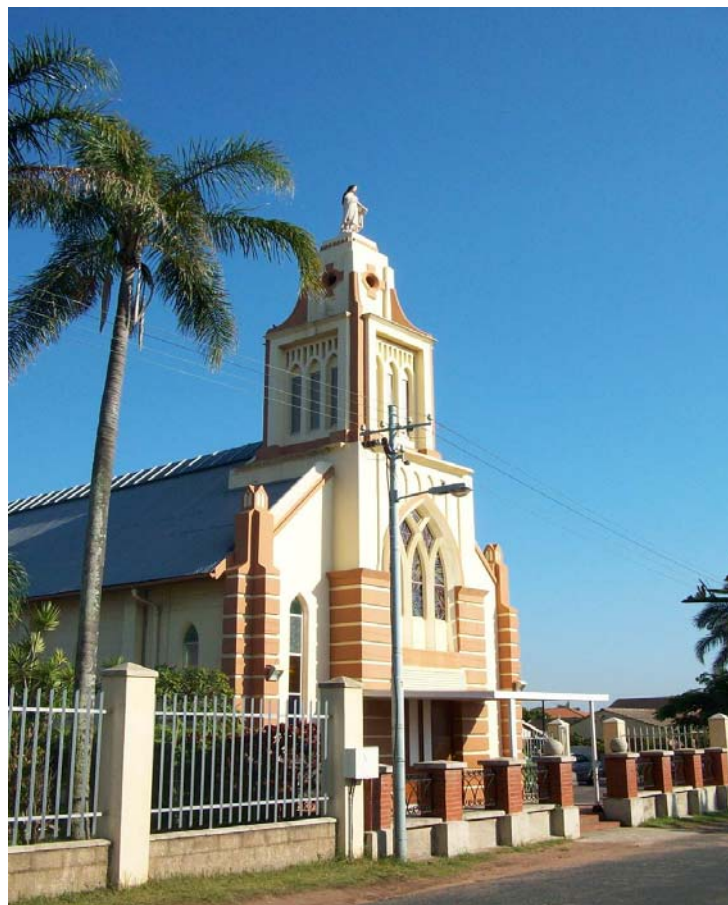
Figure 8: St. Theresa's Catholic Church
