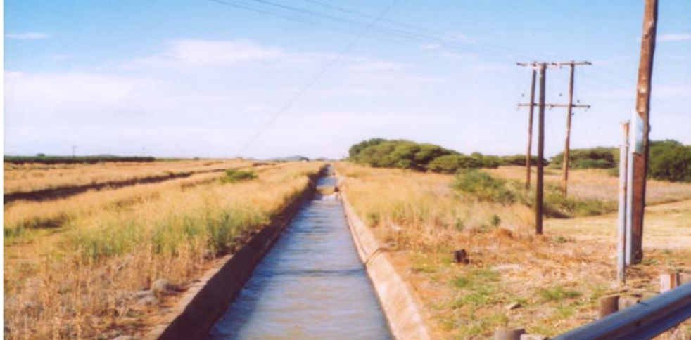
Photo 6. 1 Main irrigation canal system used for water distribution at Riet River Irrigation Scheme
