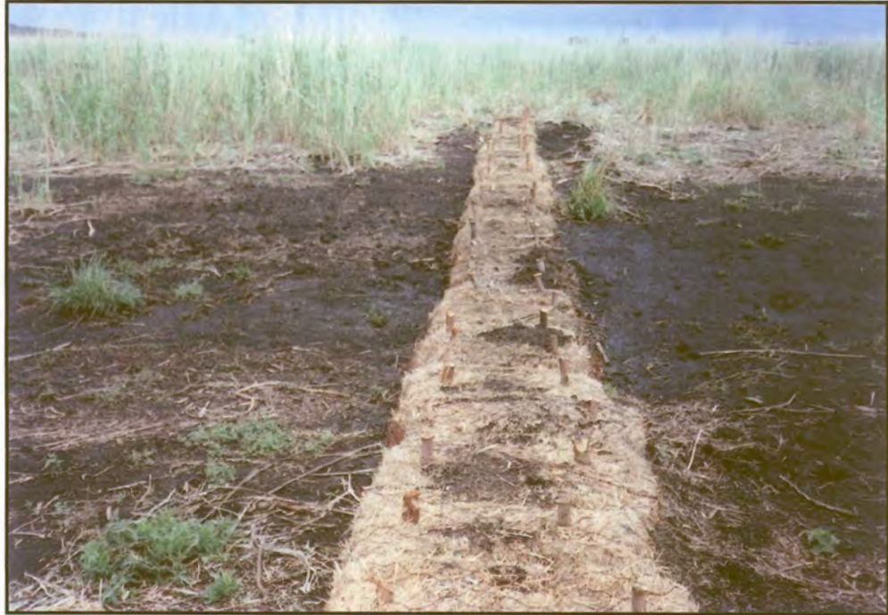
Figure 2: Grass bales used at the Rietvlei wetland.
