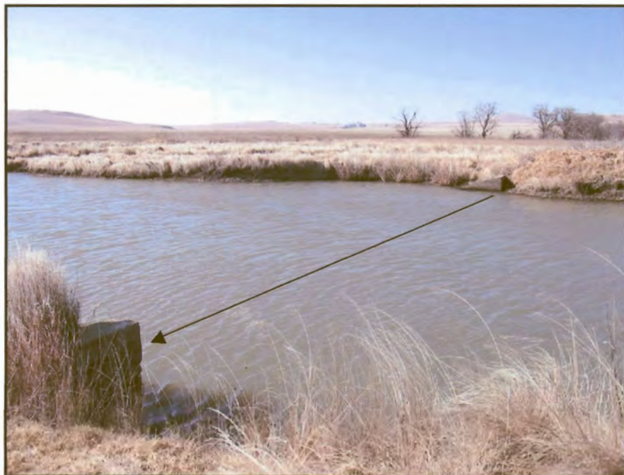
Figure 48: Site no. 4. Merel's vlei. A small weir drowned below the water surface.
