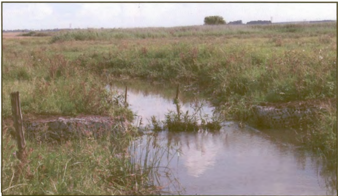
Figure 84: A drowned gabion structure between sites no. 6.1 and 6.2 due to an increase in back flooding from the structure at site no. 6.3.
