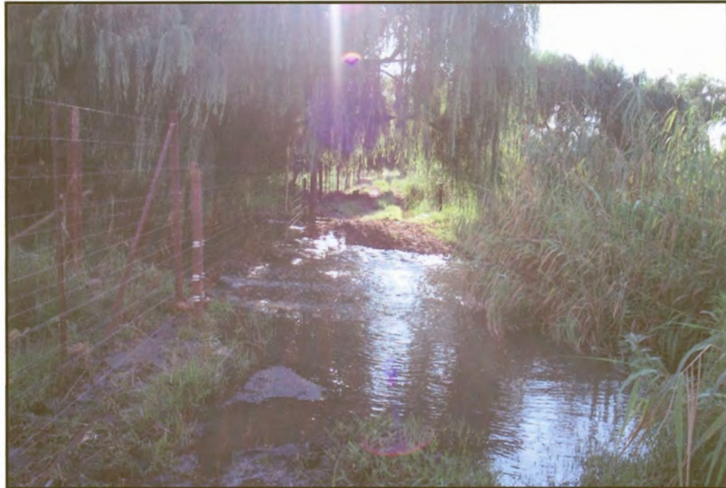
Figure 71: Site no. 1. A man-made drift was built across the entry point into the Rietvlei Nature Reserve. Due to this the flow of water has been concentrated.
