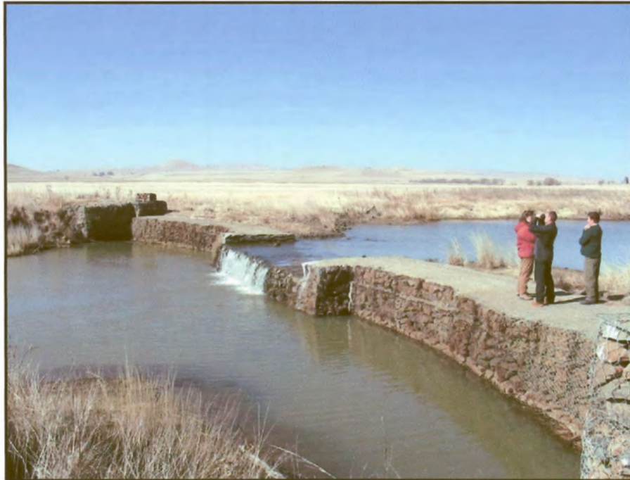
Figure 49: Site no. 5. Gabion structure.
