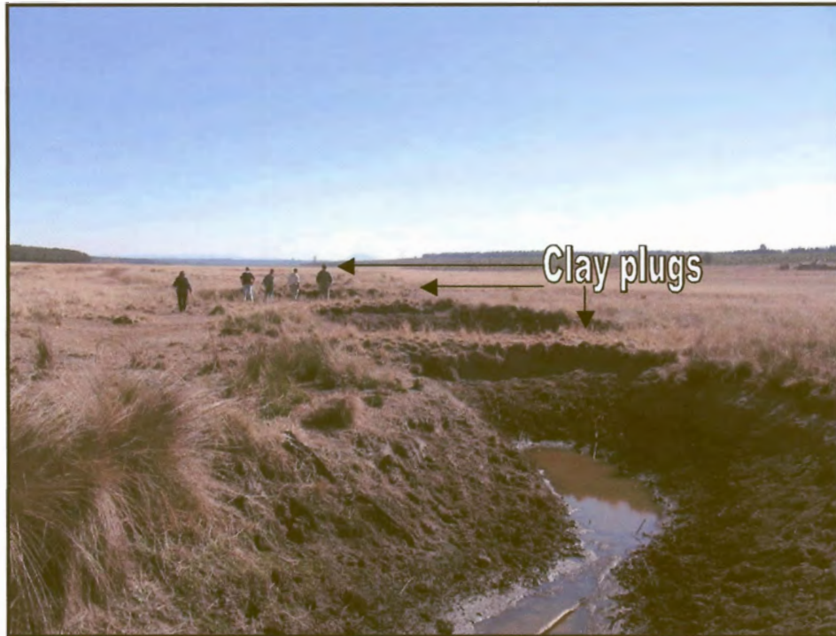
Figure 58: Site no 1: Clay plugs in a badly eroded channel at the northern border with private owners.
