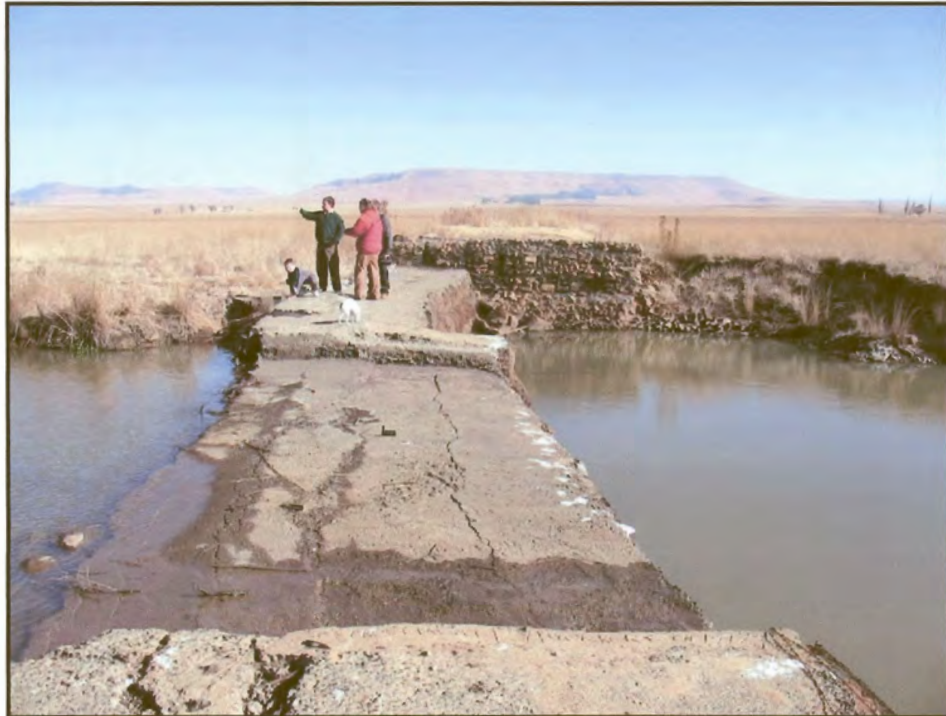
Figure 47: Site no. 3. Merel's vlei. The gabion structure was constructed in 1997/8. Measures were put in place to try and stabilise the bank erosion.
