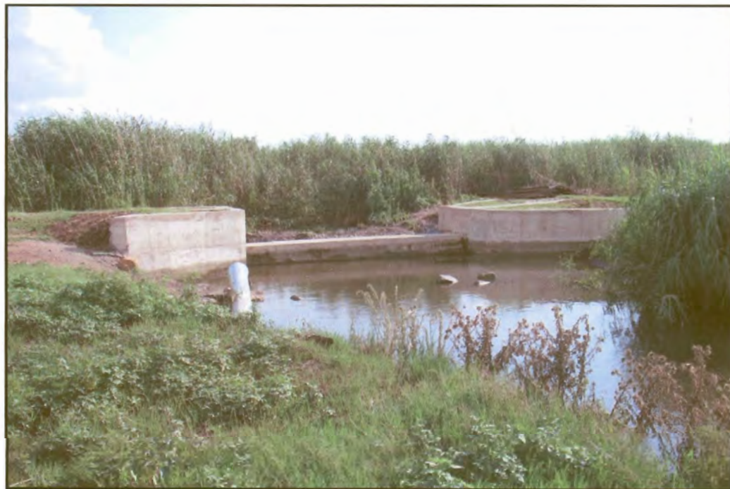
Figure 76: Site no. 4. Eroded culverts on the road crossing were replaced by a concrete weir.
