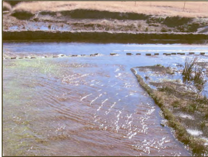
Figure 10: Geocell lining at the Wilge wetland structure.
