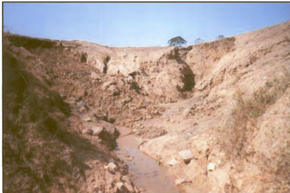
Figure 30: Uvova site damage to chute preparation after July 2002 floods (Photo: M. Astrup).
