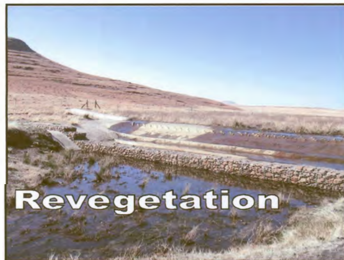
Figure 14: Bioengineering at the Wilge wetland structure.
