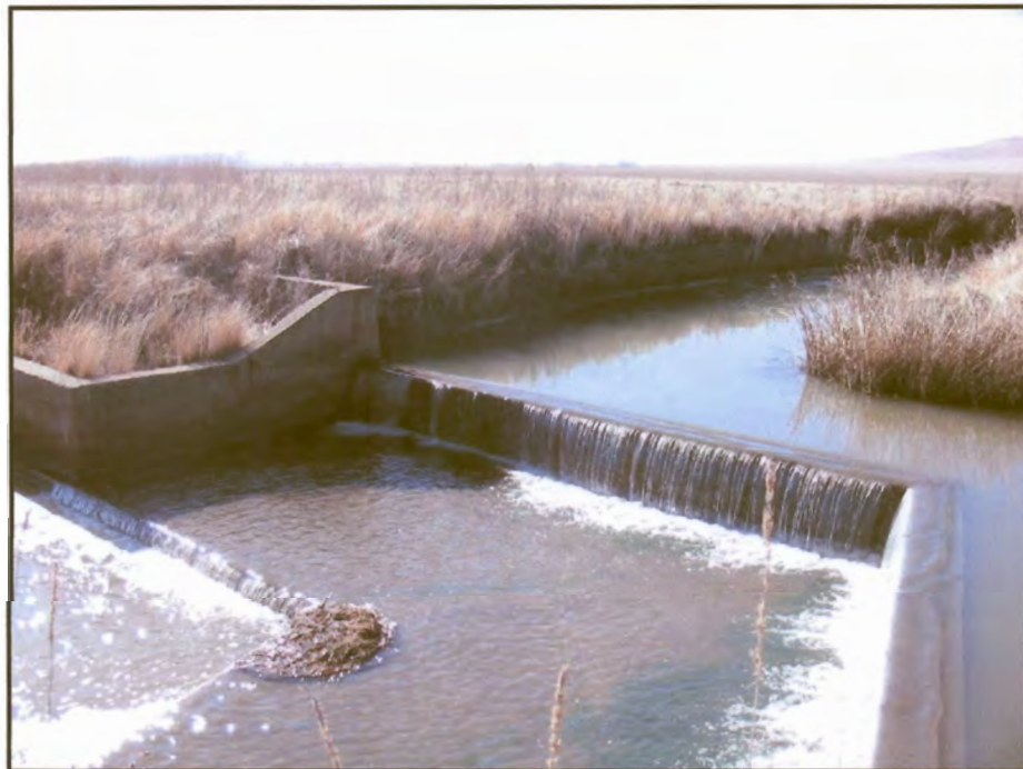
Figure 44: Site no. 1. Concrete weir.
