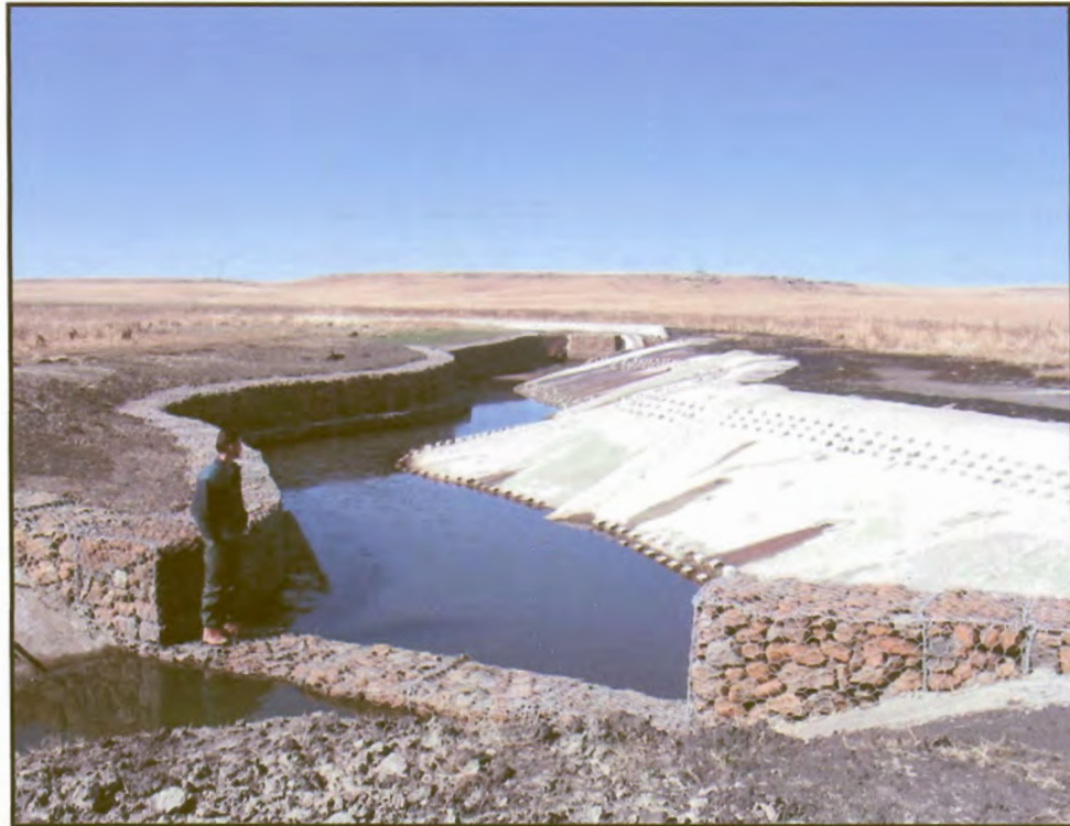
Figure 38: Close up of the headcut rehabilitation structure.
