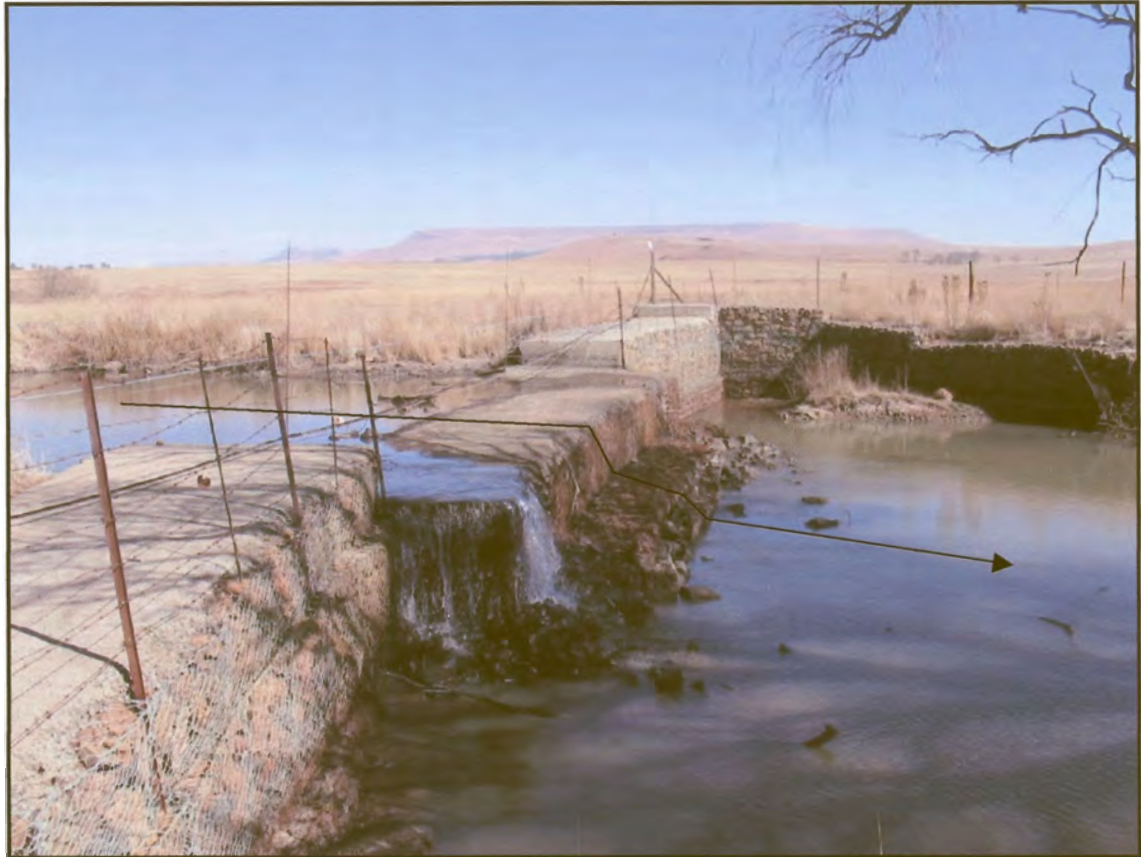
Figure 51: Site no. 7. The Northern border of the Seekoeivlei Nature Reserve. A gabion structure was constructed in the flow of the Klip River to promote the flooding of the floodplain and to raise the water table.
