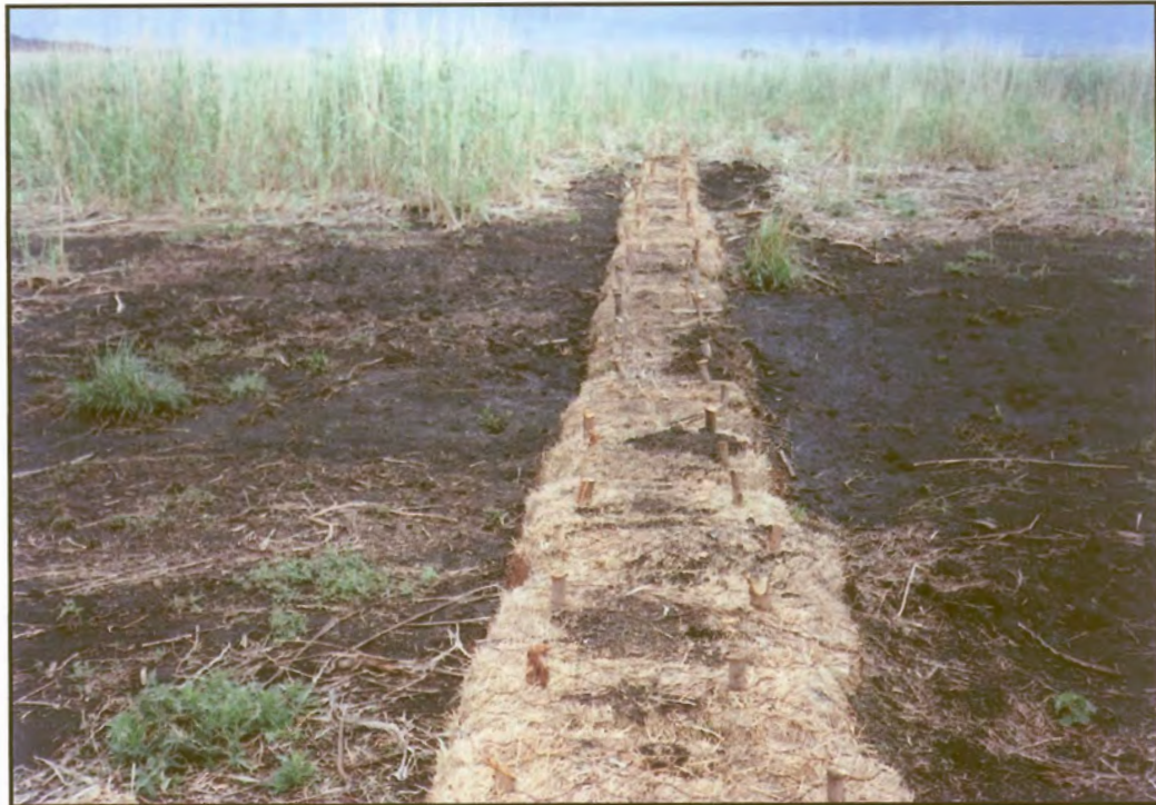
Figure 73: At site no. 2.1 the shallow erosion gully was stabilized with grass bales.
