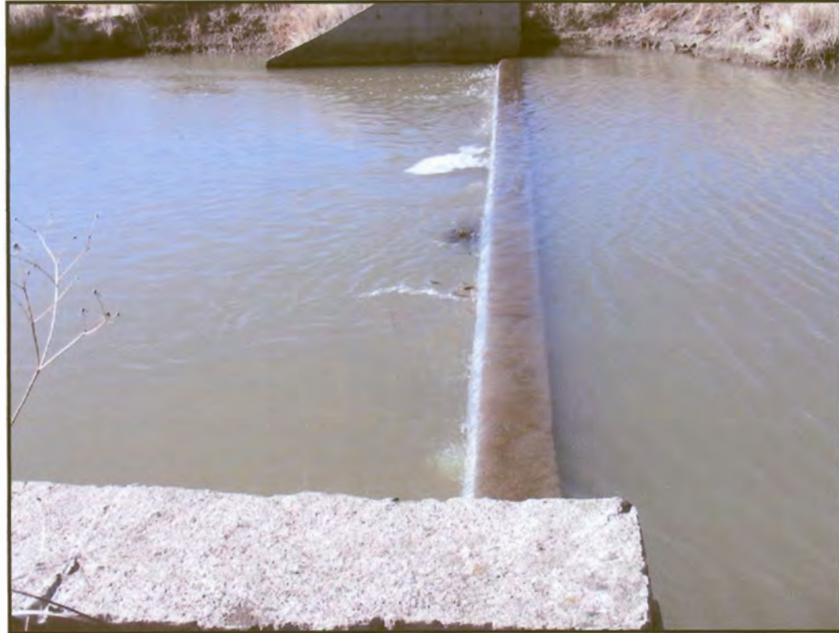
Figure 45: Site no. 2. Concrete weir.
