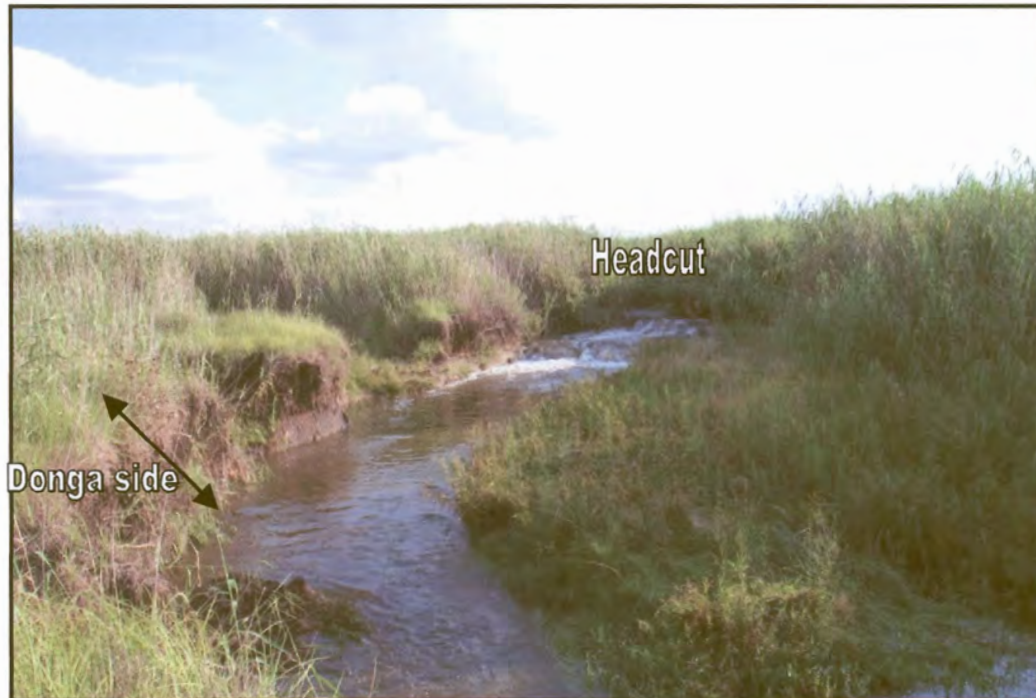
Figure 75: Headcut and donga (incised drainage channel) at site no. 3.1. The donga sides need to be sloped and re-vegetated.
