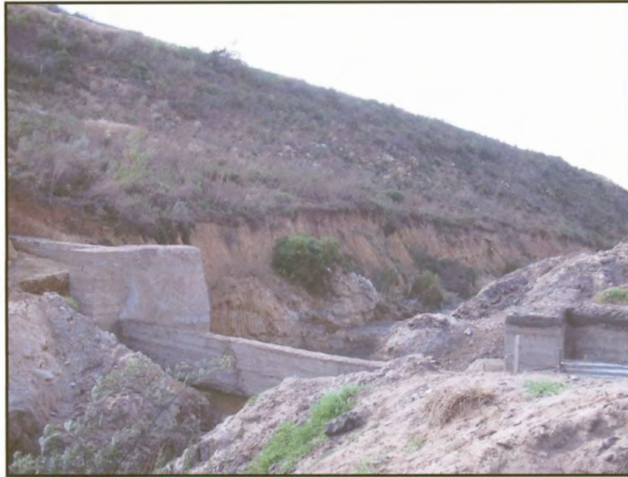
Figure 14: Rehabilitation structure 3: Concrete Weir being constructed.
