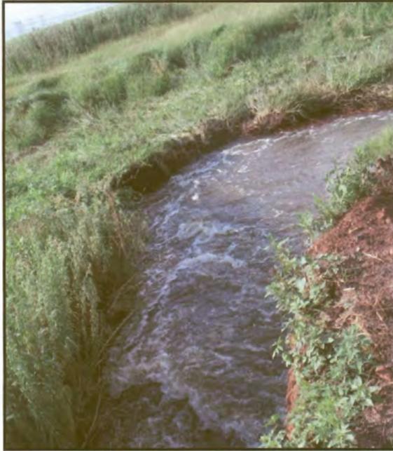
Figure 77: Site no. 4. A bypass furrow used during the construction of a concrete weir in the causeway was blocked to prevent channel erosion.
