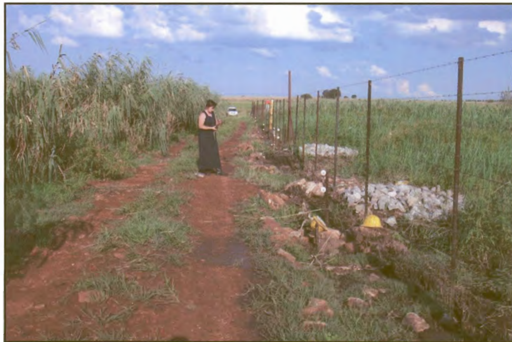
Figure 72: Site no. 1. Energy dissipaters were constructed along the drift to spread the flow and dissipate the energy.
