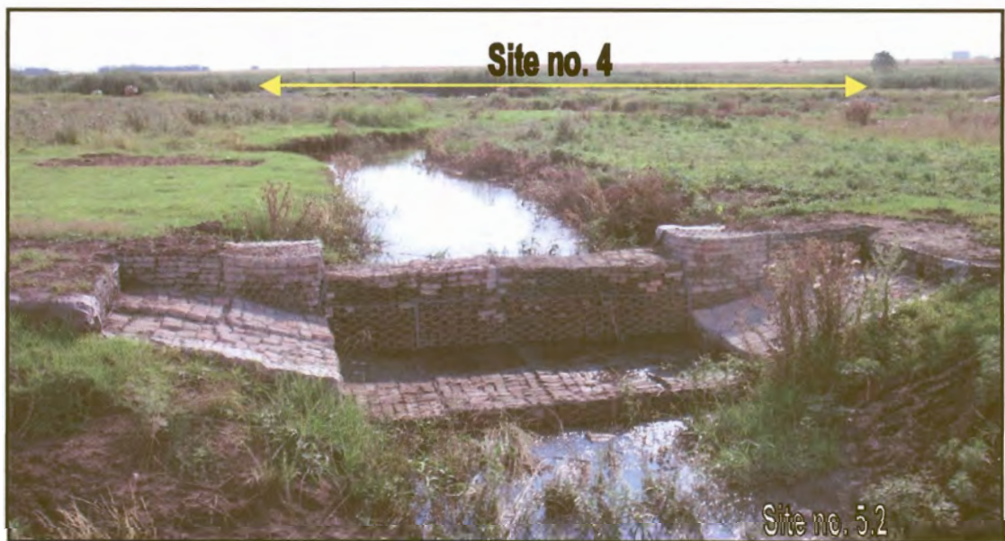
Figure 82: Gabion structure at site no. 5.2. Note the difference in the water table upstream and downstream of the structure.
