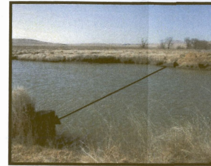
Figure 100: Site 4 at Merel's vlei. The weir is drowned below the water surface.
