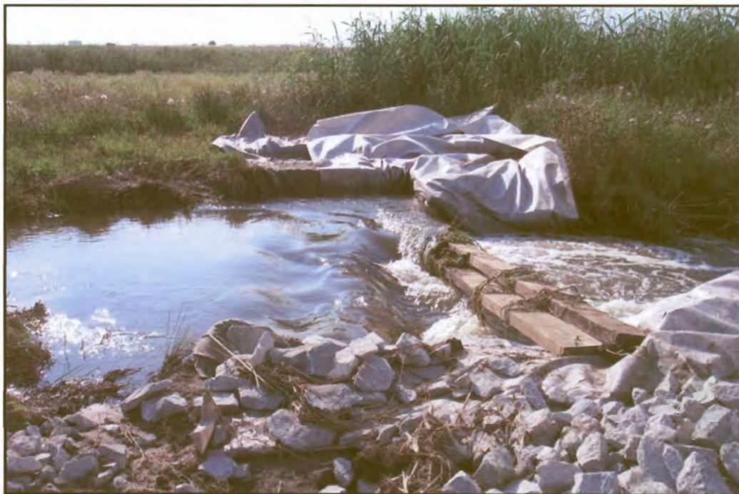
Figure 80: Construction of a gabion in progress at site. no. 5.1.1. Flooding is taking place.
