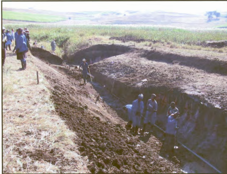
Figure 27: Before flooding. Photo taken up stream on 4 July 2002 at the Amatigulu site.
