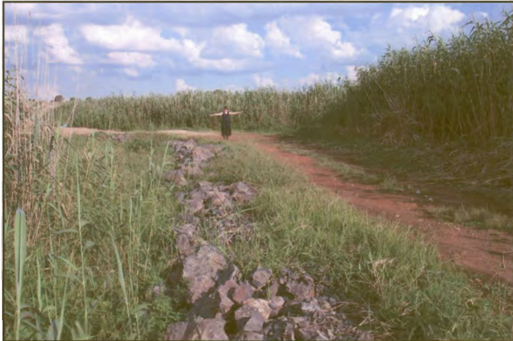
Figure 78: Site no. 4. A causeway was applied as a structure to disperse water and to raise the water level in the wetland. Downstream of the structure the erosion was stabilised by using rock packs.
