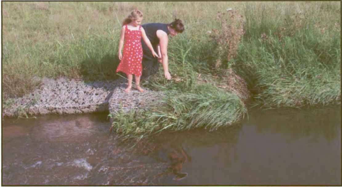
Figure 83: Site no. 6.1. Note the higher water table behind the structure. The bent grass on the bank of the channel indicates a previous flooding event.
