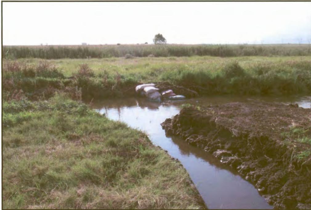
Figure 79: Site no. 5.1. A bypass furrow has been constructed to allow the construction of a gabion weir to facilitate the raising of the water table and to disperse the water.
