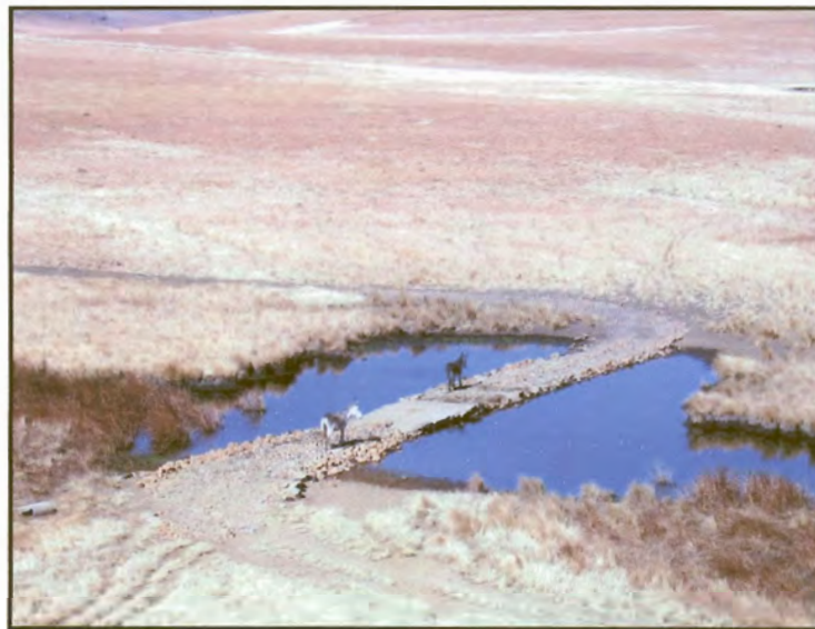
Figure 36: Road crossing downstream of the rehabilitation structure.
