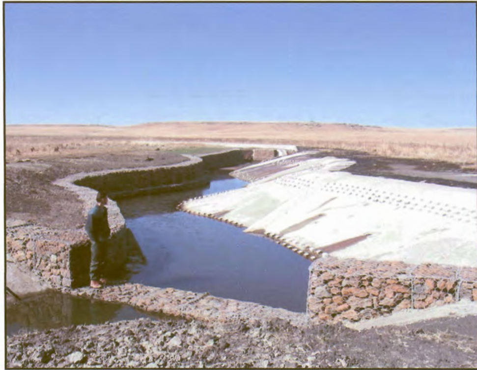
Figure 38: Close up of the headcut rehabilitation structure.
