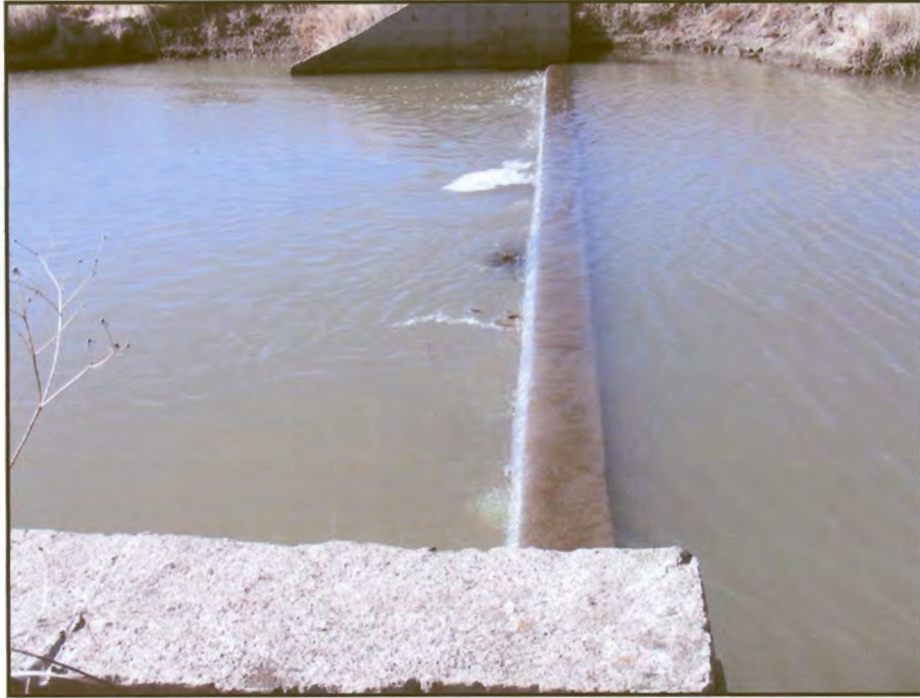
Figure 45: Site no. 2. Concrete weir.
