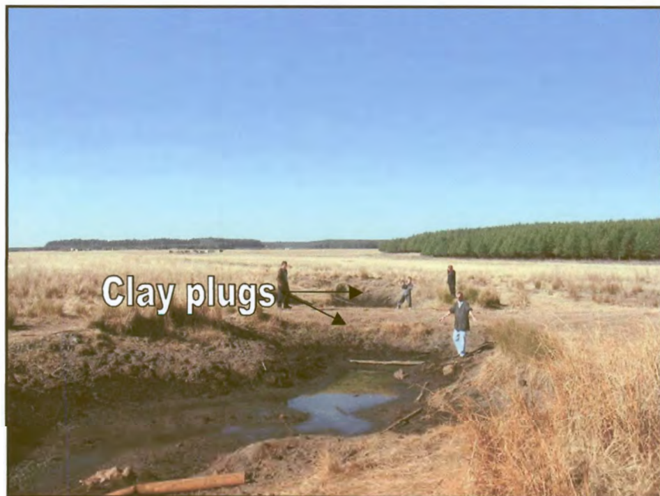
Figure 63: Site no. 5: Main drain with smaller drains along the side. Clay plugs act like dam walls.
