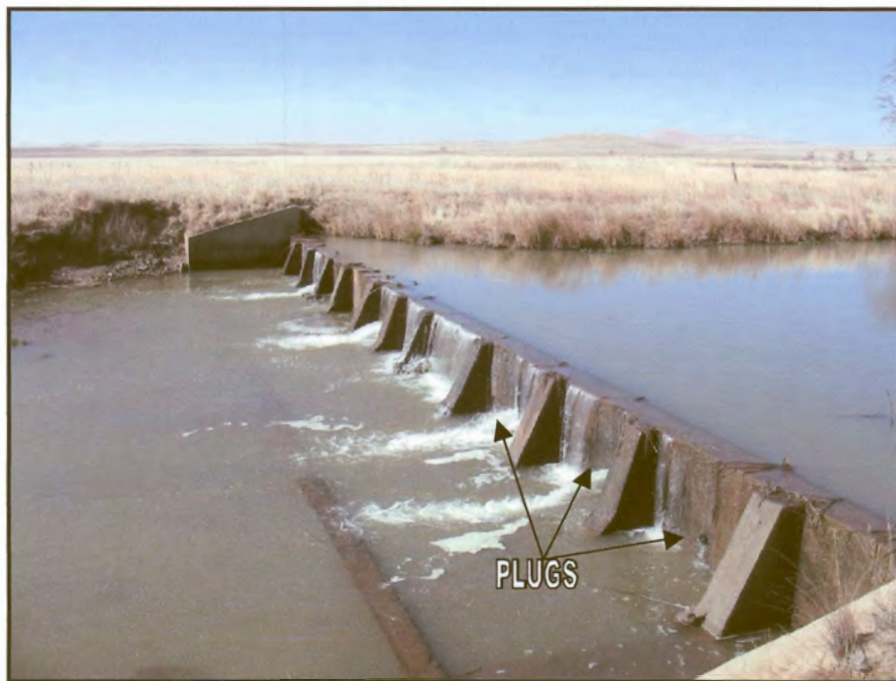
Figure 50: Site no. 6. The work involved lifting the existing structure higher, strengthening the structure and closing the drain holes (1997). Note that most of the plugs have been washed out.
