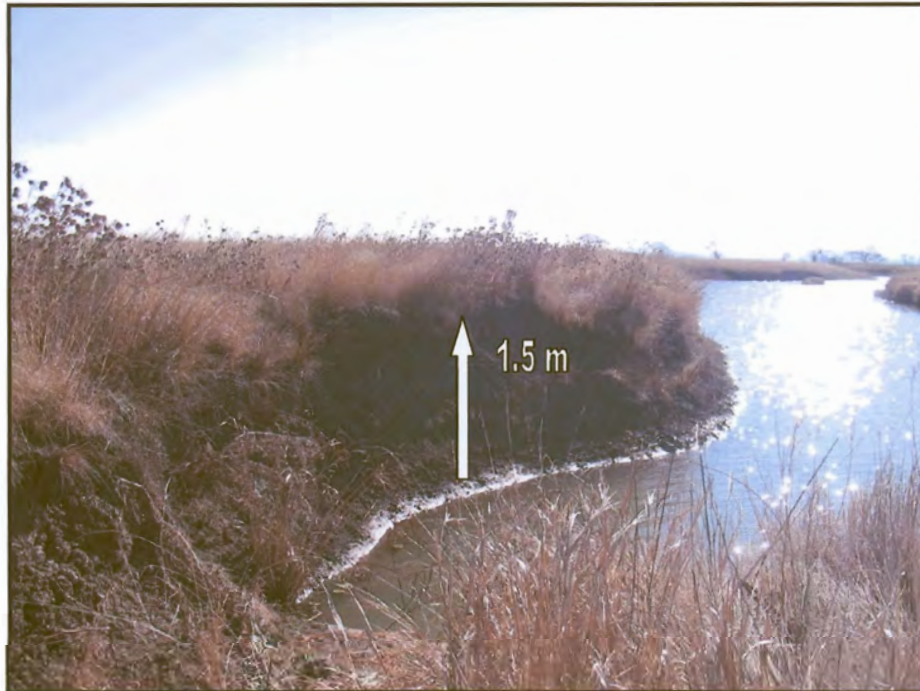
Figure 46: Site no. 2. Bank erosion.
