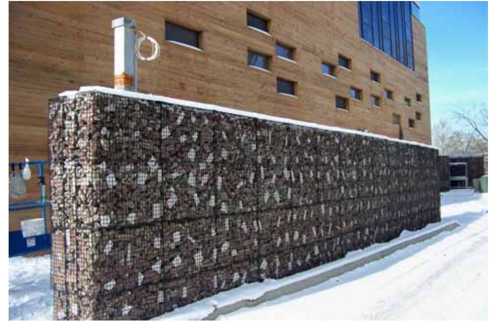
figure 146. re-used brick gabion perimeter wall
