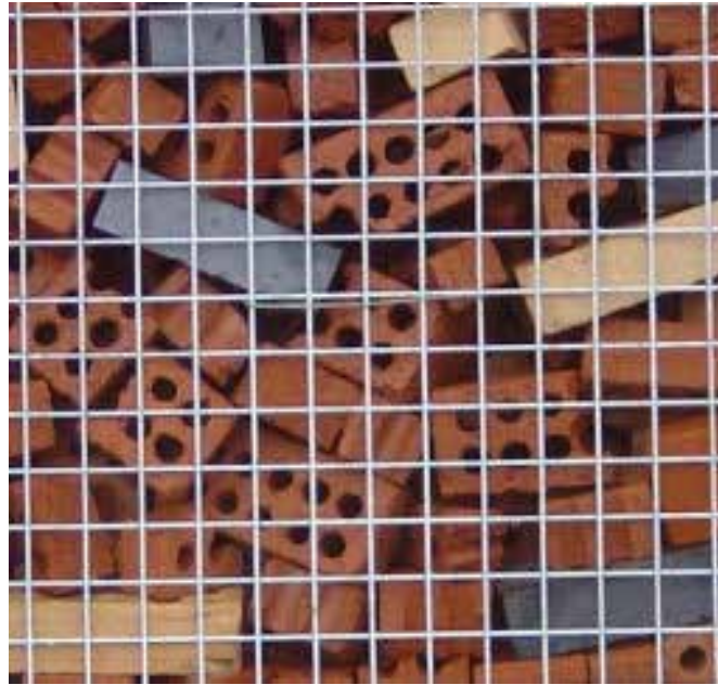
figure 147. example of re-used brick gabion wall
