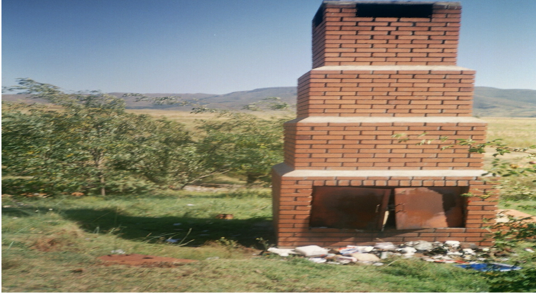
Figure 5.15: Incinerator used to store and treat waste at Malealea Health centre
