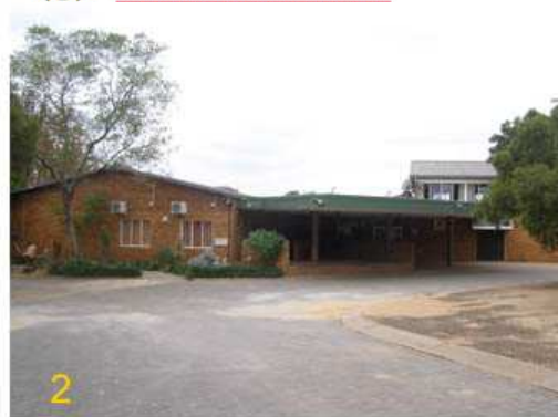
Figure 42. Main entrance of New Hope School building
