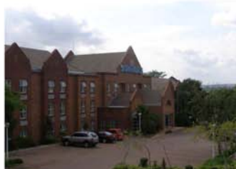
Figure 31. City town lodge, Atterbury road
