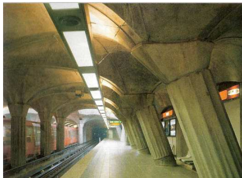
Figure 92. Skylight indicate the direction of movement
