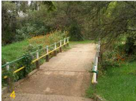
Figure 44. Existing bridge over Waterkloof spruit on interior road towards sport grounds
