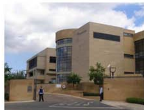
Figure 30. New Investec offices
