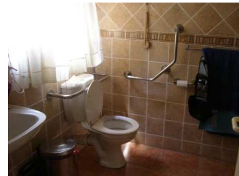
Figure 110. Grab rail for toilet layout
