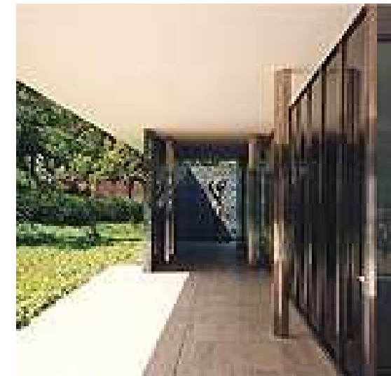
Figure 77. Steel column and glass facade
