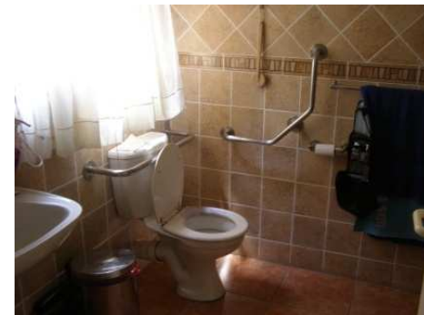
Figure 110. Grab rail for toilet layout
