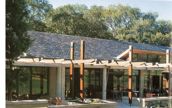
Figure 72. View towards restaurant area
