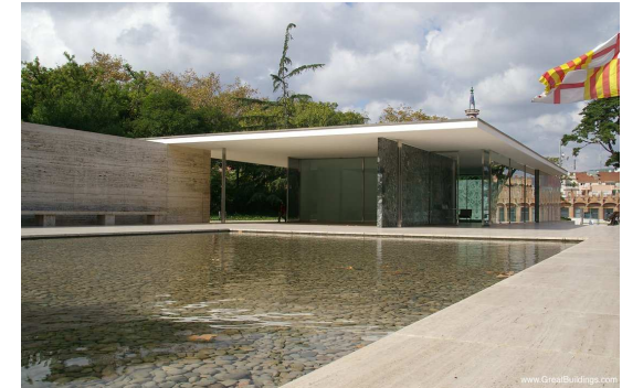
Figure 76. Elevation over pond
