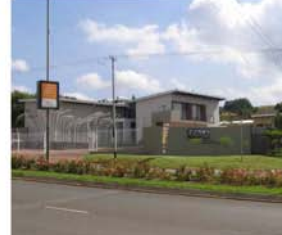
Figure 32. Attitude office park, Atterbury road
