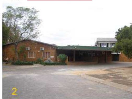
Figure 42. Main entrance of New Hope School building
