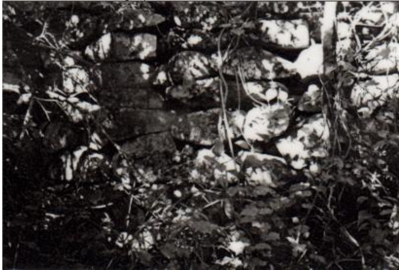
MUDZIMUNGALE: another cleared space
