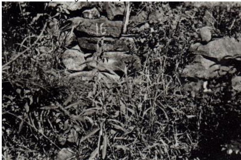
DZATA RUINS - Foundations
