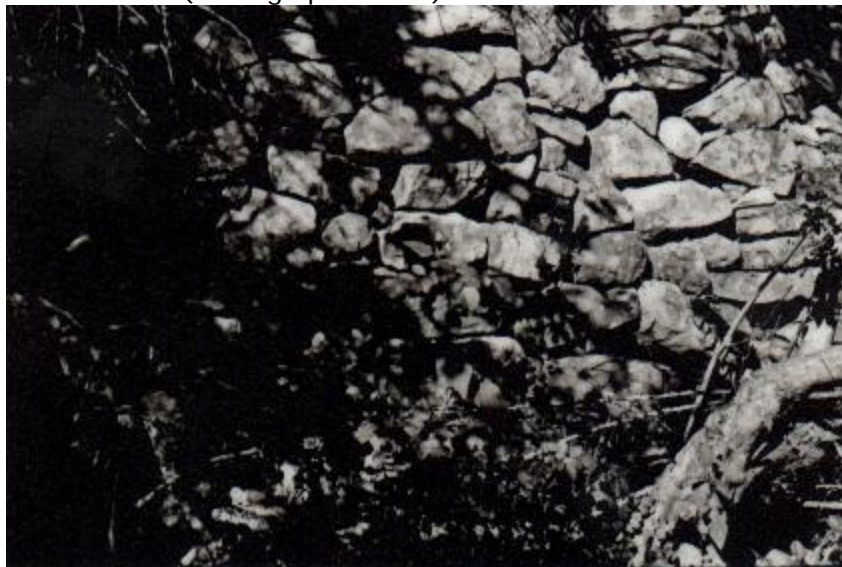
DZATA RUINS – An old wall repaired according to the new style of building (top right corner)
