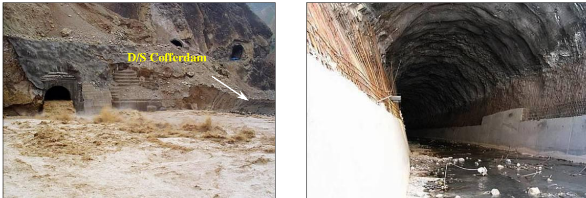
Figure 5.3.1. The diversion tunnel at outlet and down stream coffer dam, during the heavy flood 2006 (left). Diversion tunnel with temporary support elements. The final reinforced concrete lining has been done in the lower part of tunnel (right).
